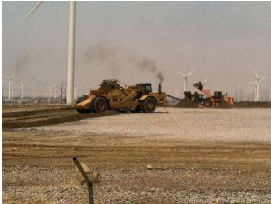
Figure 6. Yard close-out activities at the Devers 2 Yard.
