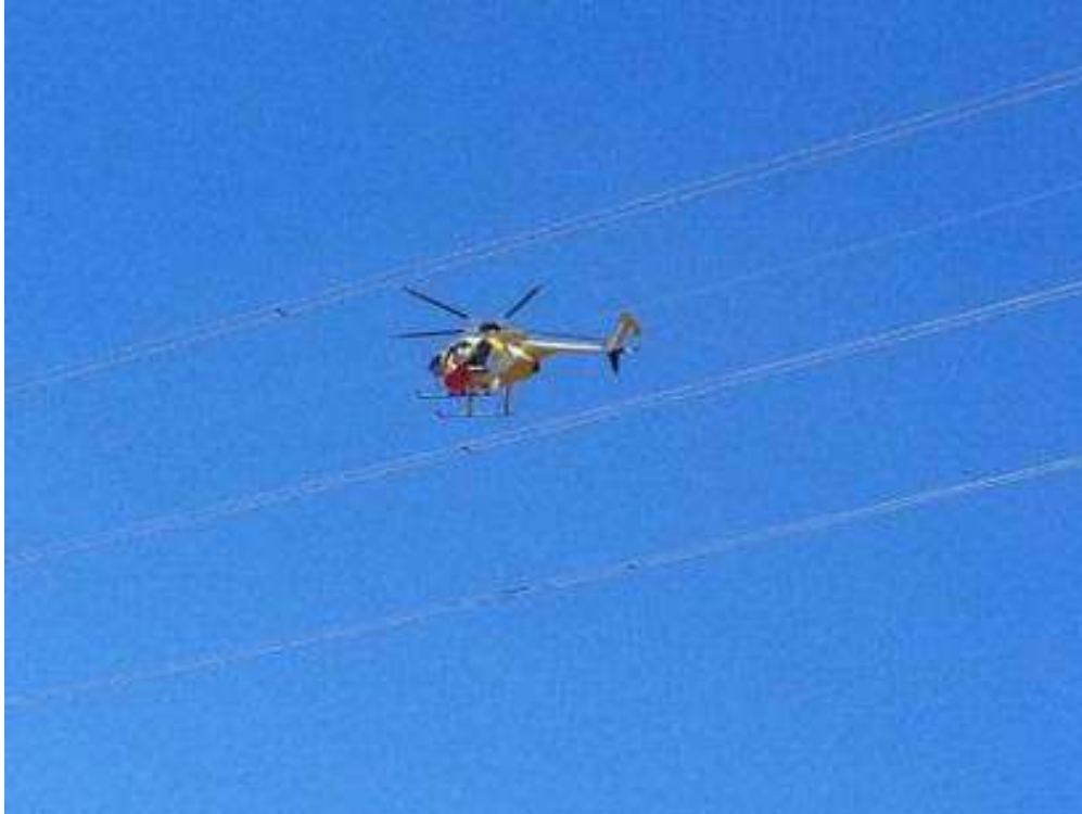
Figure 1. Marker ball installation between Towers 1111 and 1112.
