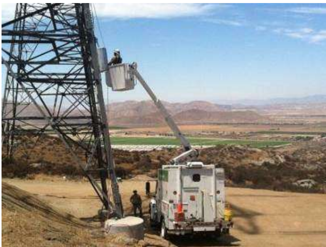
Figure 3. Telecommunication splicing work at Tower 1128.
