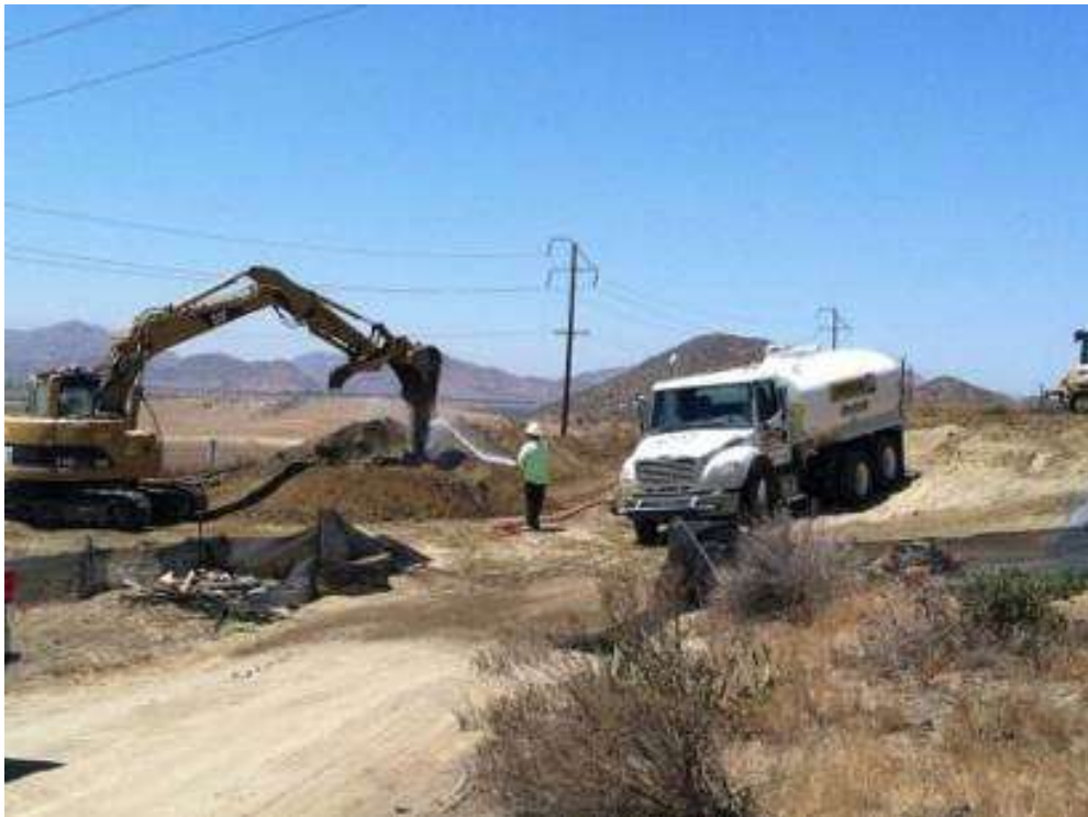
Figure 2. Site stabilization activities at Tower 1114.
