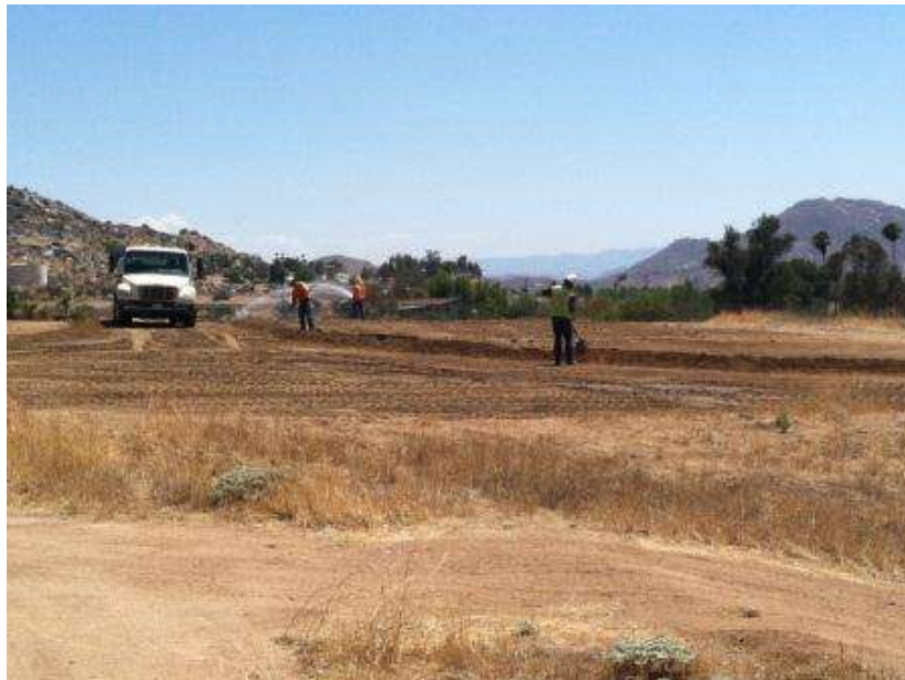
Figure 3. Site Stabilization activities at Tower 1146.
