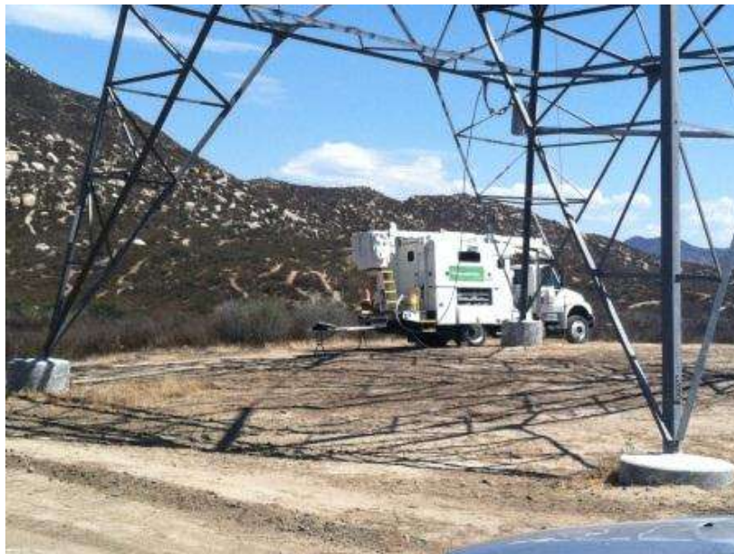
Figure 4. Telecommunication splicing activities at Tower 1094.
