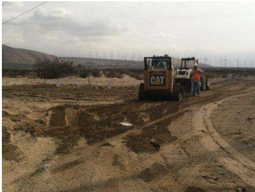
Figure 3. Site stabilization activities at Tower 1029.
