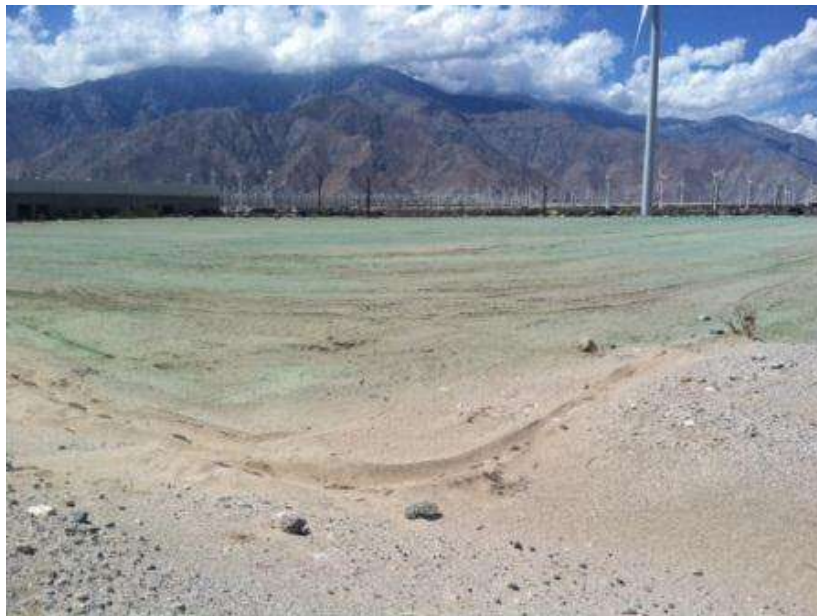
Figure 4. Soil stabilizer applied to the Devers 2 Yard.
