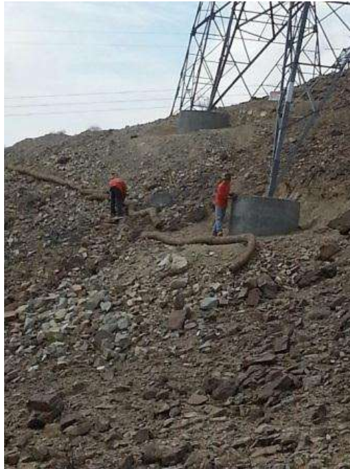
Figure 1. BMP removal at Tower 2310 (photo courtesy of FRED).
