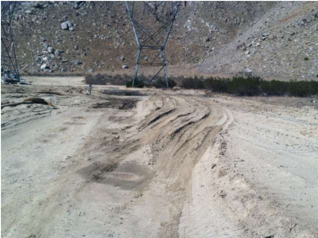
Figure 3. Tracks leading of the main access road near Tower 1031.
