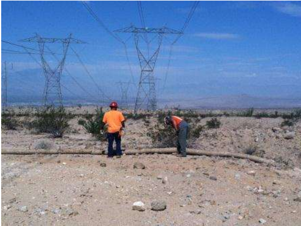
Figure 1. BMP removal at Tower 2265.
