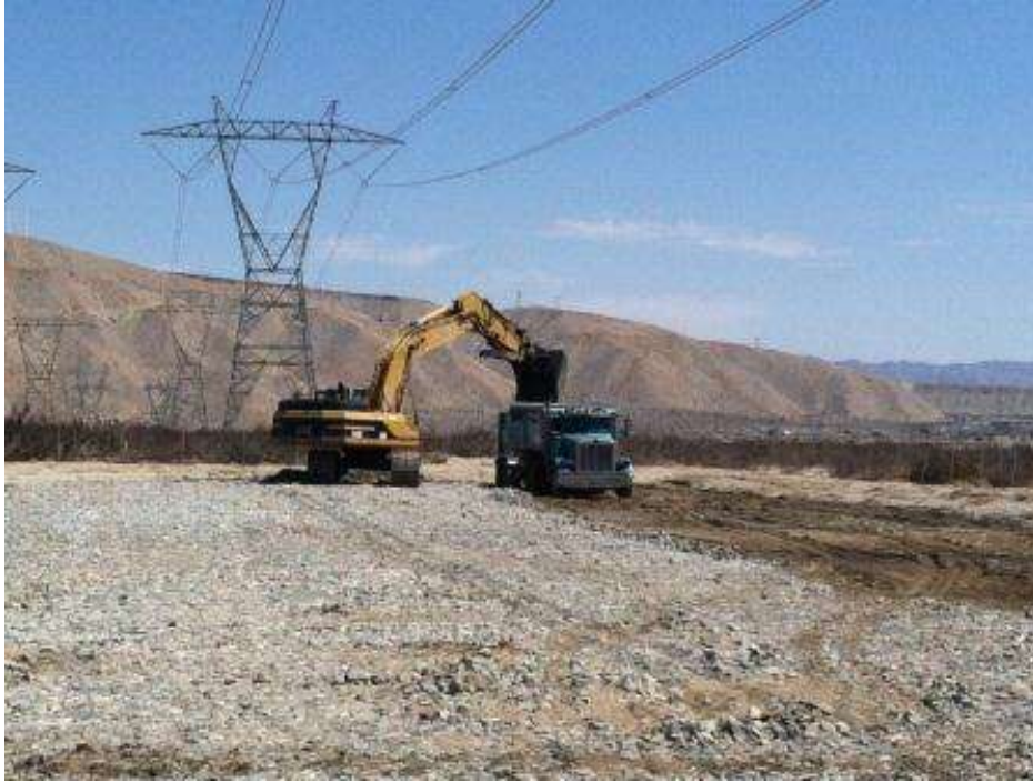
Figure 1. Removal of gravel at HLZ-H1A during site stabilization activities.
