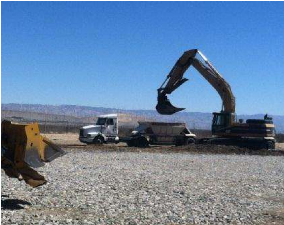
Figure 2. Gravel removal as part of site stabilization activities at HLZ H1X.
