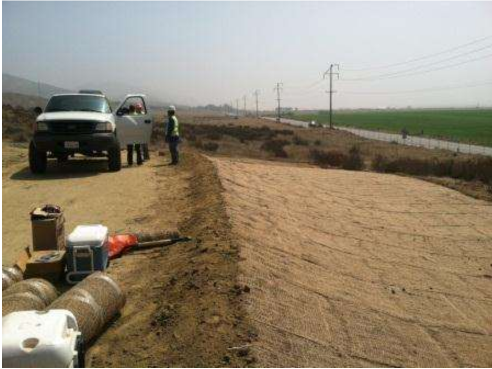
Figure 1. Jute netting installation at Tower 1114.
