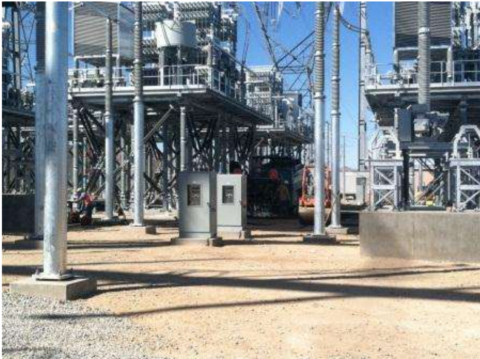
Figure 3. Paving activities at the Series Capacitor.
