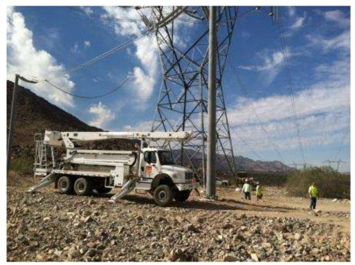
Figure 2. Construction crews setting up to remove the Transposition Tower near DPV2 Tower 2526.
