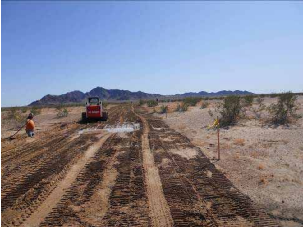
Figure 3: Development of the “drive and crush” road leading to the CRS site.
