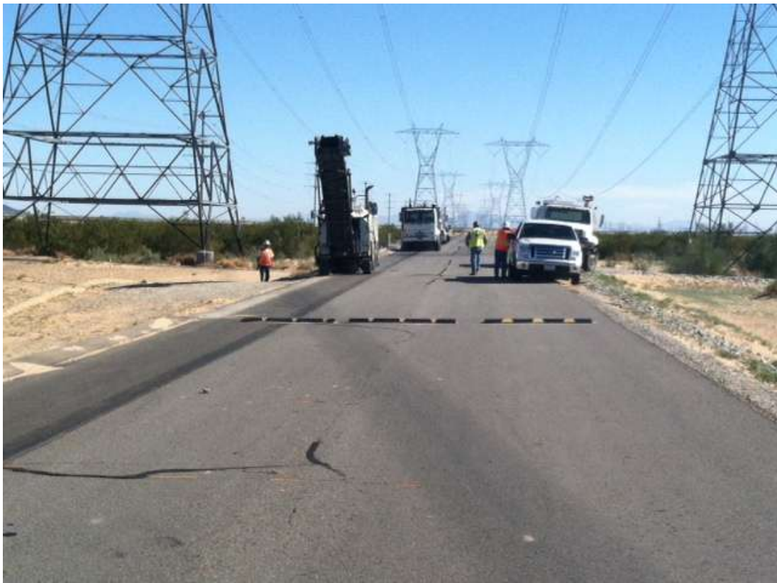
Figure 3. Repairs to the CRS access road.
