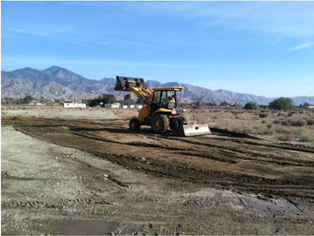
Figure 1. Site scarification activities in preparation for hydroseeding at Tower 1062.
