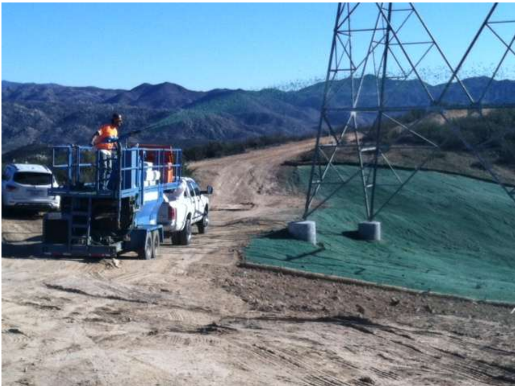
Figure 2. Hydroseeding at Tower 1096.
