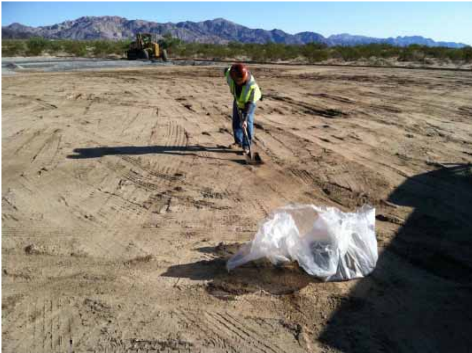
Figure 2: Soil from small oil leak being removed and placed within a spill kit at the Summit Construction Yard.
