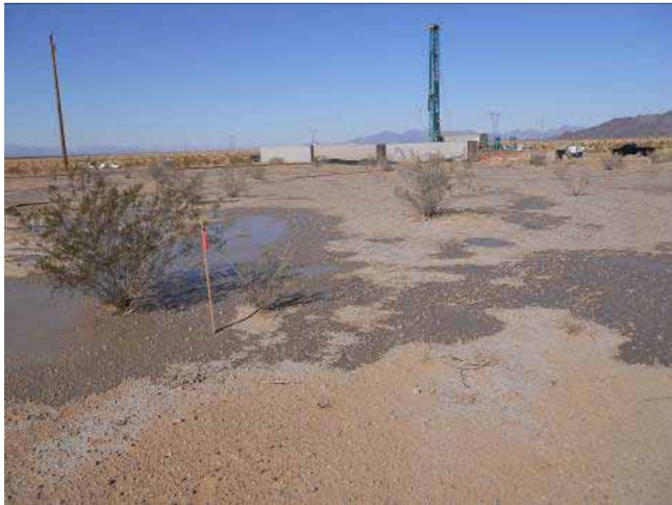
Figure 6: Surface spreading of zone-testing release water at CRS. Note water line set up in background.
