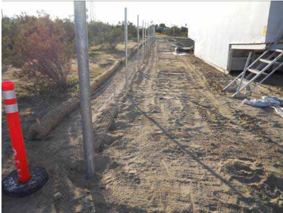
Figure 1: Installation of desert tortoise exclusionary fencing at the Summit Construction Yard.
