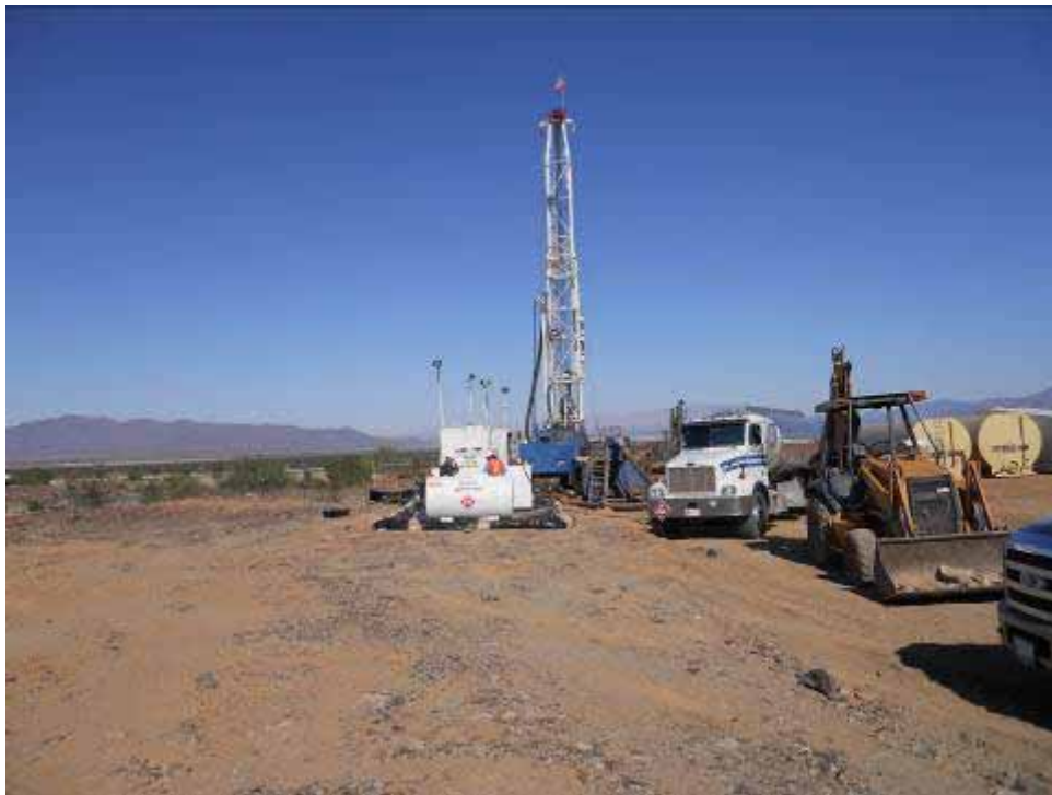
Figure 8: Drill rig erected and operational at Red Bluff Substation site.
