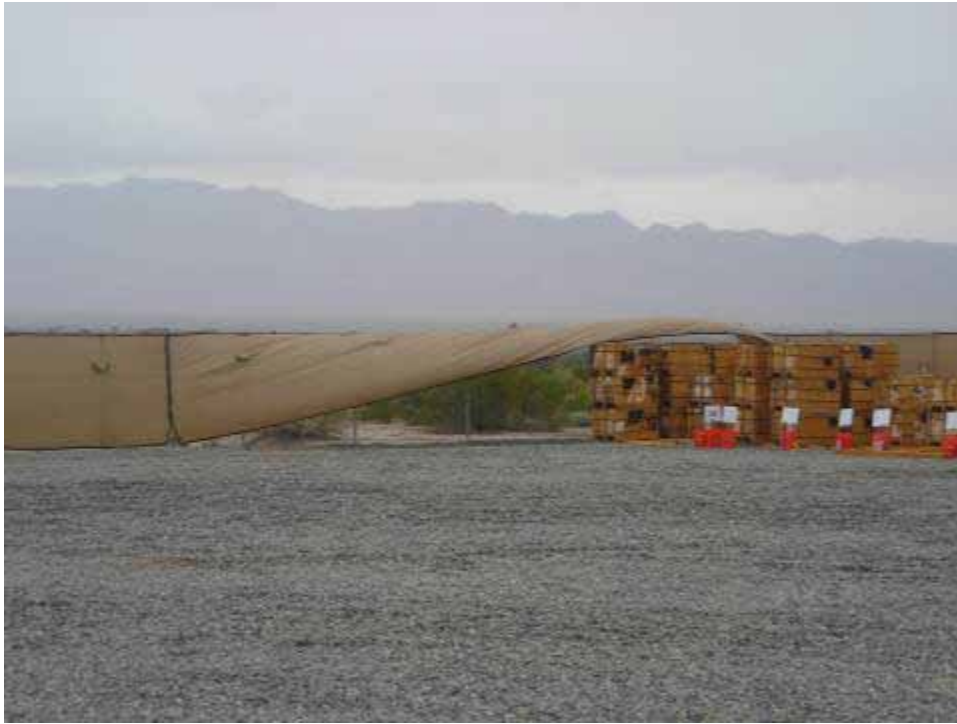
Figure 1: High winds resulting in minor damage to the fencing and privacy screening at the Desert Center #1 Construction Yard.
