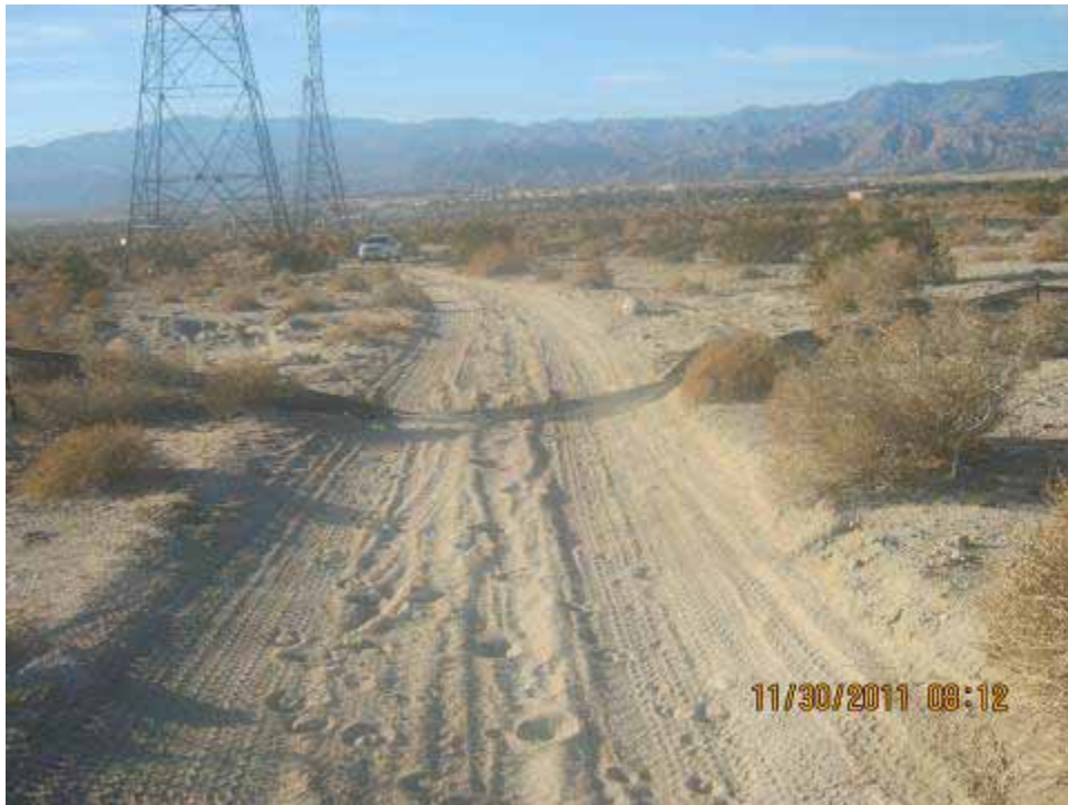
Figure 2: View along stub road of damaged exclusionary fencing at Tower #2132.
