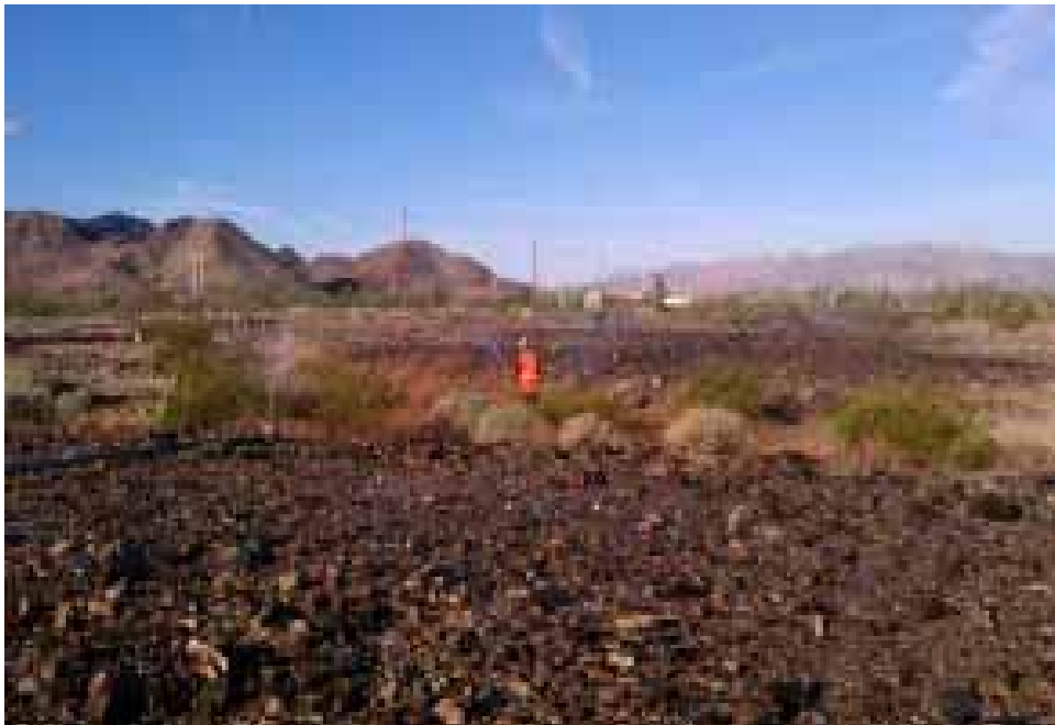
Figure 6: Surface release of water through the sprinkler system installed at Red Bluff Substation site.
