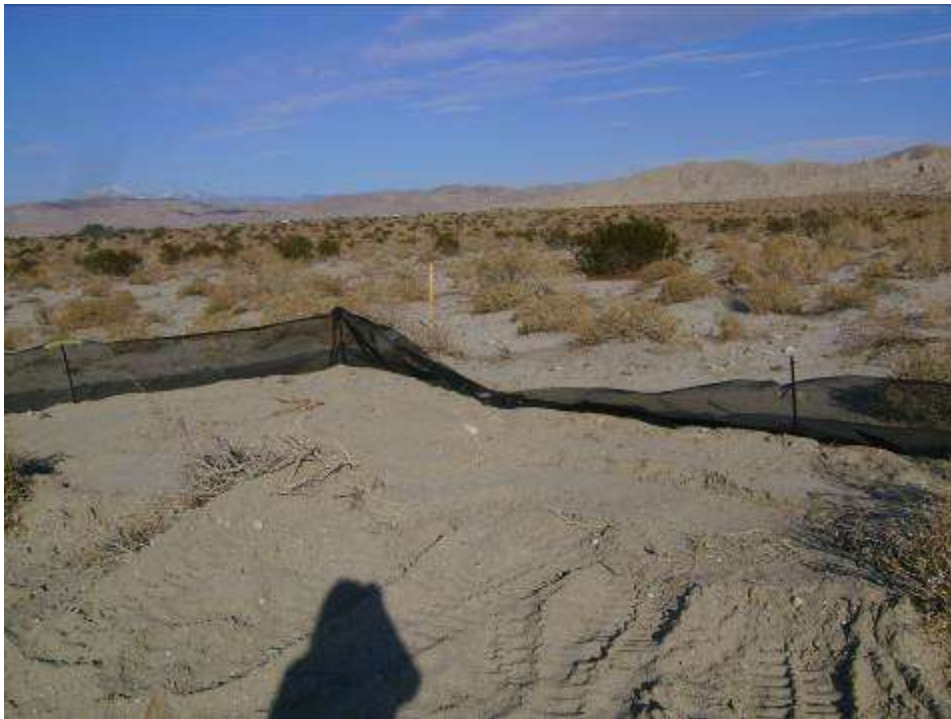
Figure 4: Damaged exclusionary fencing at Tower #2133 that had not yet been repaired by the subject period.
