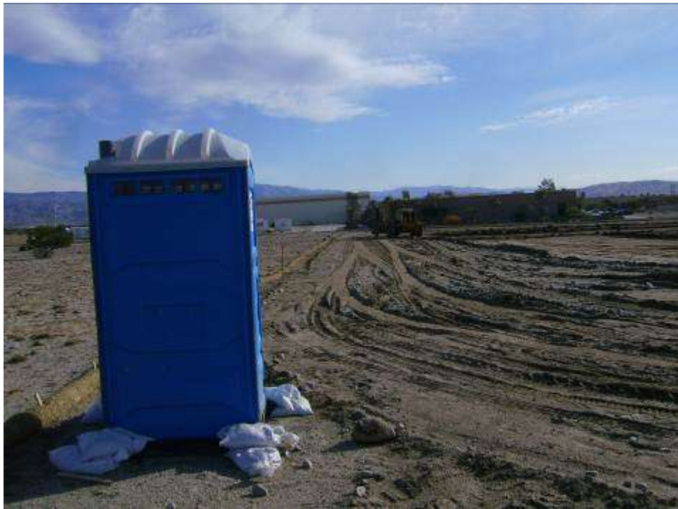
Figure 5: BMPs installed and grubbing activities occurring at the Devers #2 Construction Yard.
