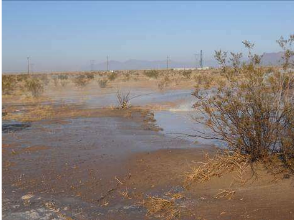
Figure 7: Surface water release activities and potential for pooling water at the CRS site documented by CPUC EM on December 19.
