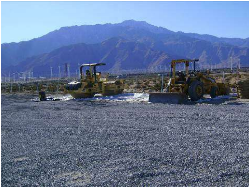
Figure 6: Heavy equipment stage on plastic sheeting at the Devers #2 Construction Yard.
