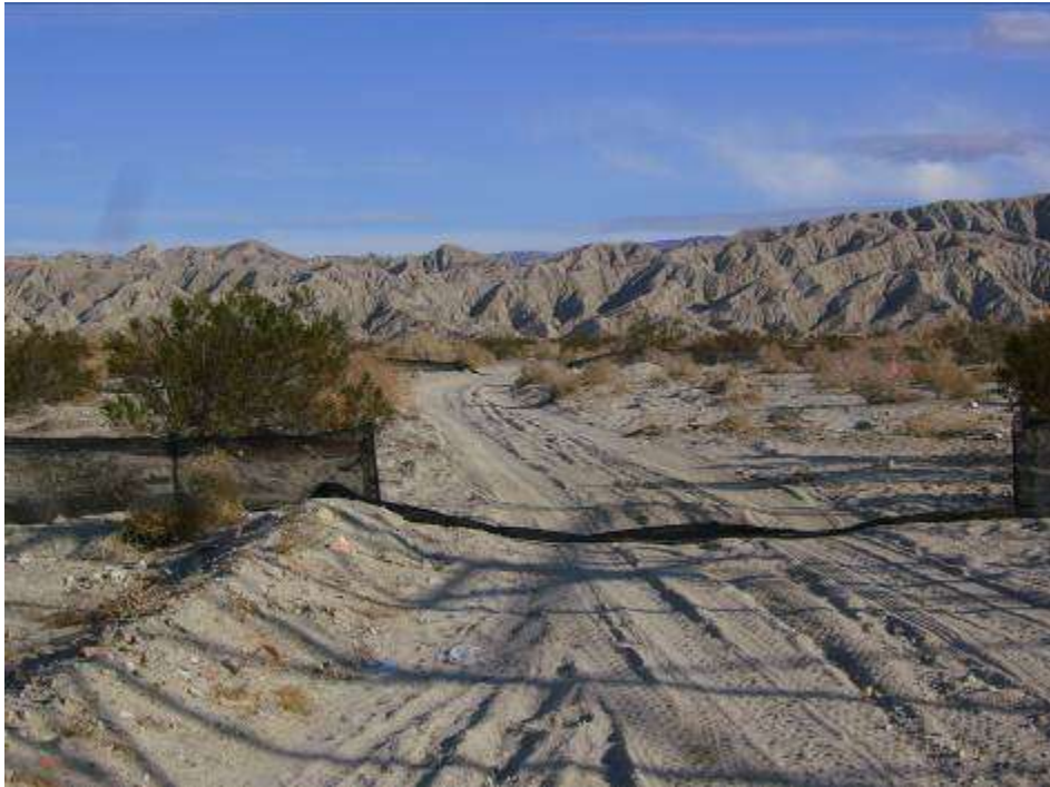
Figure 3: Damaged exclusionary fencing at Tower #2132 that had not yet been repaired by the subject period.
