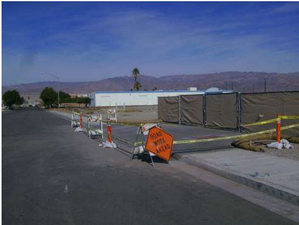
Figure 3: Completion of the driveway at the Indio #2 Construction Yard.
