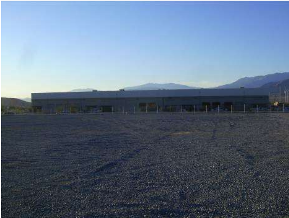
Figure 1: Completion of fence installation at the Devers #2 Construction Yard.
