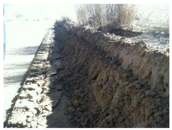
**Figure 5.** Road berms along the access road to CRS.
