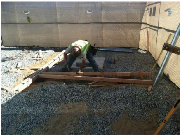
**Figure 7.** Preparation for auger drilling at the Devers Yard temporary power source. (Photo Courtesy of Dean Ritter)
