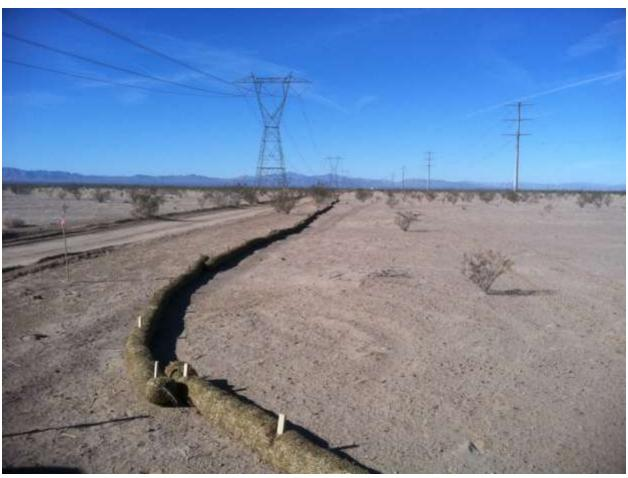
Figure 2. BMP installation along the access road to CRS from Wiley's Well Road.
