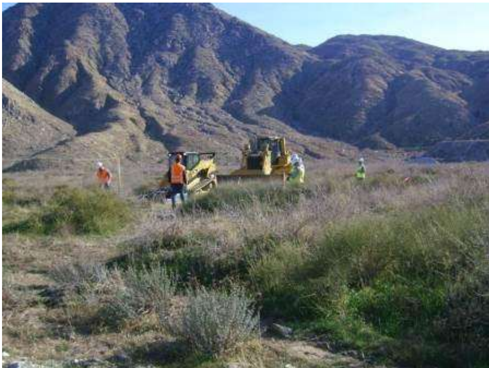
Figure 2. Setting up for vegetation clearing at Tower 1061.
