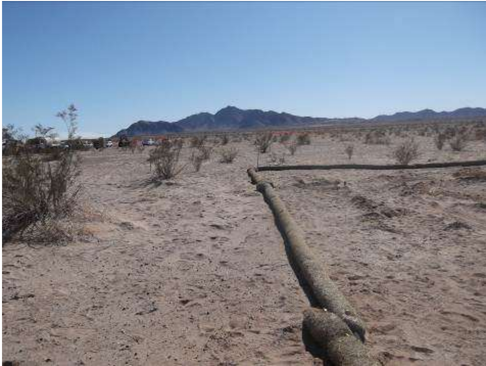
Figure 1. BMPs installed at Tower CR1-2W
