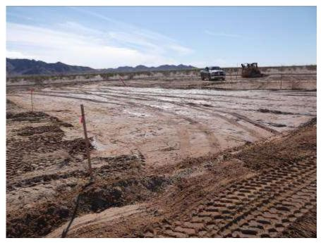
**Figure 1.** Grading activities completed at Tower CR1-2E.
