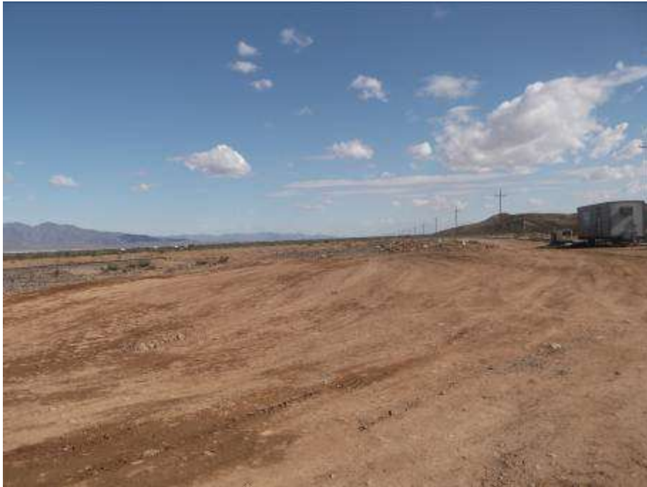
Figure 8. View east from southwest corner of the Red Bluff Substation site where vegetation clearing had occurred.
