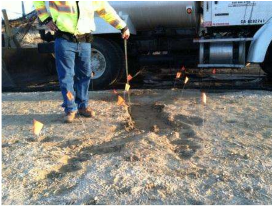
Figure 5. Diesel spill from theft of fuel from water truck at Tower 1011. (Photo courtesy of Dean Ritter).
