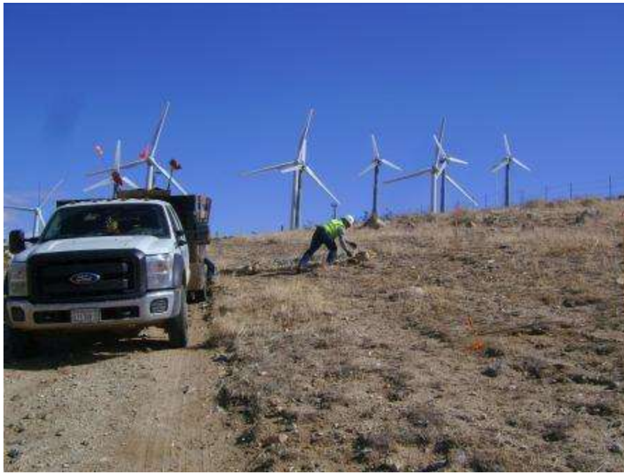
Figure 3. BMP installation at Tower 1013.
