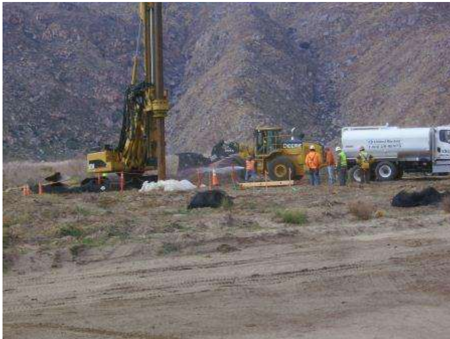
Figure 2. Foundation drilling at Tower 1061.
