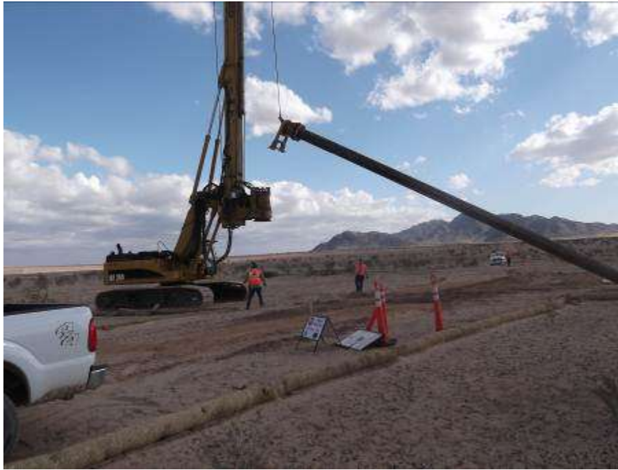
Figure 1. Preparation for drilling activities at Tower CR3-1W.
