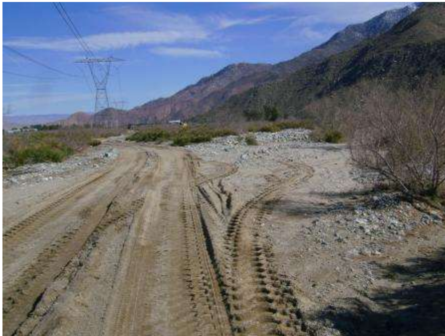
Figure 4. Tracks from where a front loader ventured off of the approved ROW into a jurisdictional water.
