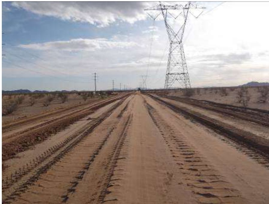
Figure 6. View east of graded primary access road at CRS.
