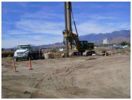
**Figure 4.** Foundation drilling at Tower R1.
