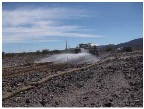
Figure 6. Fugitive dust control measures being implemented along new spur road to RB1-3E.
