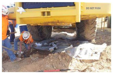
**Figure 8.** Clean up efforts for hydraulic fluid spill at Red Bluff Substation (photo courtesy of Ryan Rezek).
