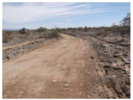
Figure 2. BMPs installed along access road associated with loop-in towers just east of Red Bluff Substation.
