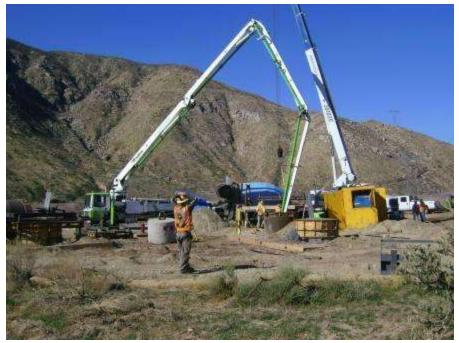
Figure 5. Concrete Pouring for foundations at Tower 1064.
