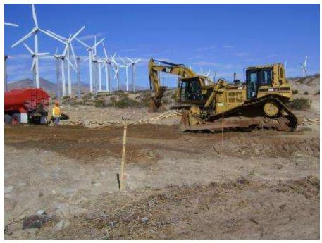
Figure 3. Spur road and crane pad grading at Tower 1016.
