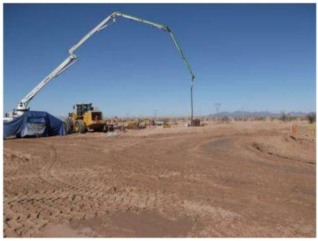
Figure 1. Foundation concrete pouring occurring at Tower CR1-2W.
