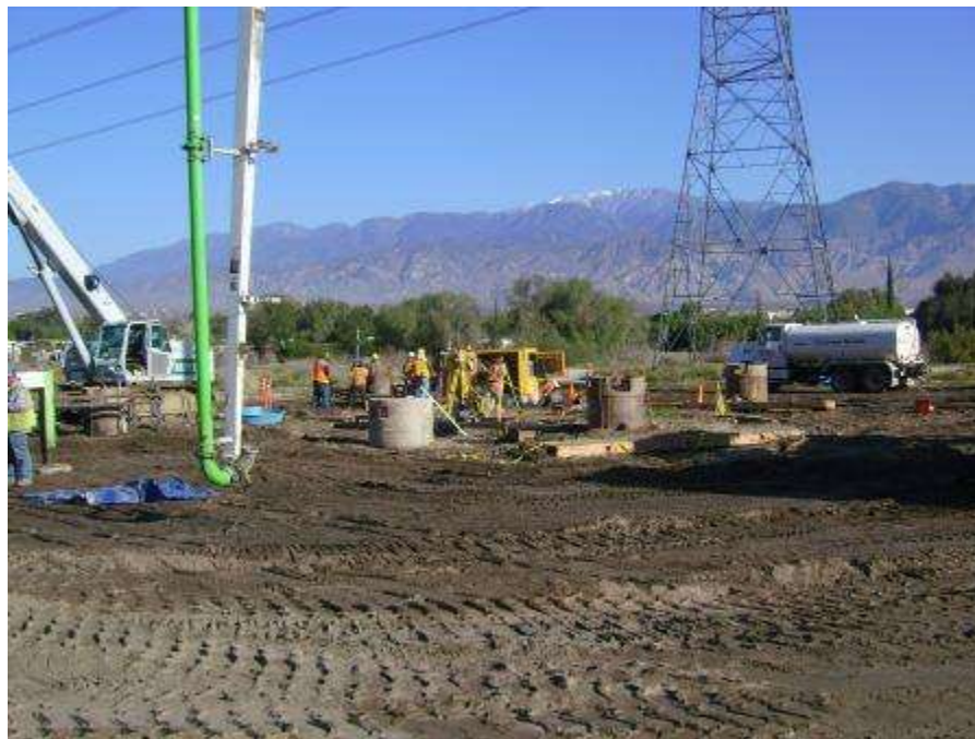
Figure 4. Foundation concrete pouring at Tower 1052.
