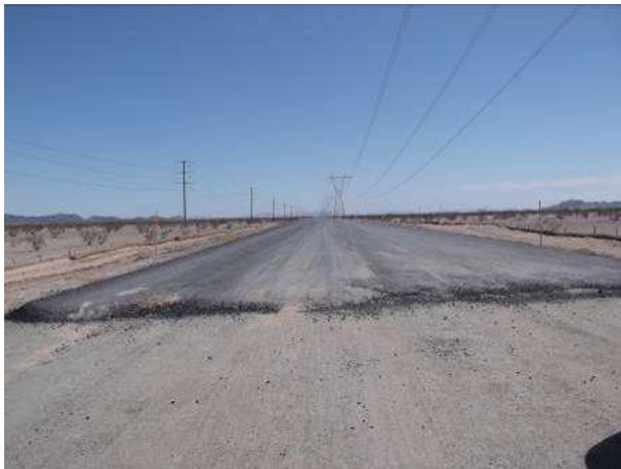
Figure 8. View east from entrance to newly paved CRS primary access road.
