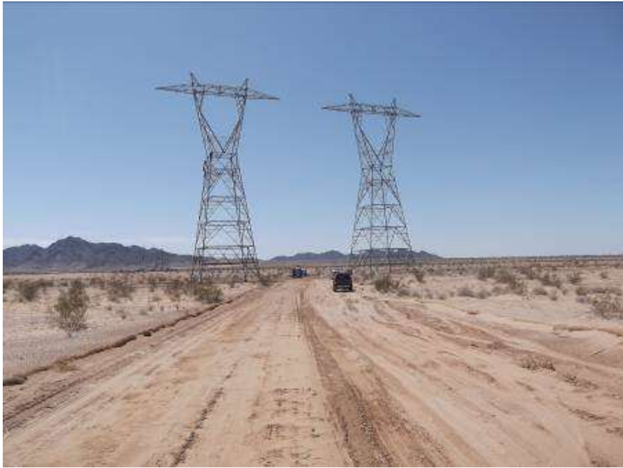
Figure 1. Assembly and erection completed at Tower 2650 and CR1-3W.
