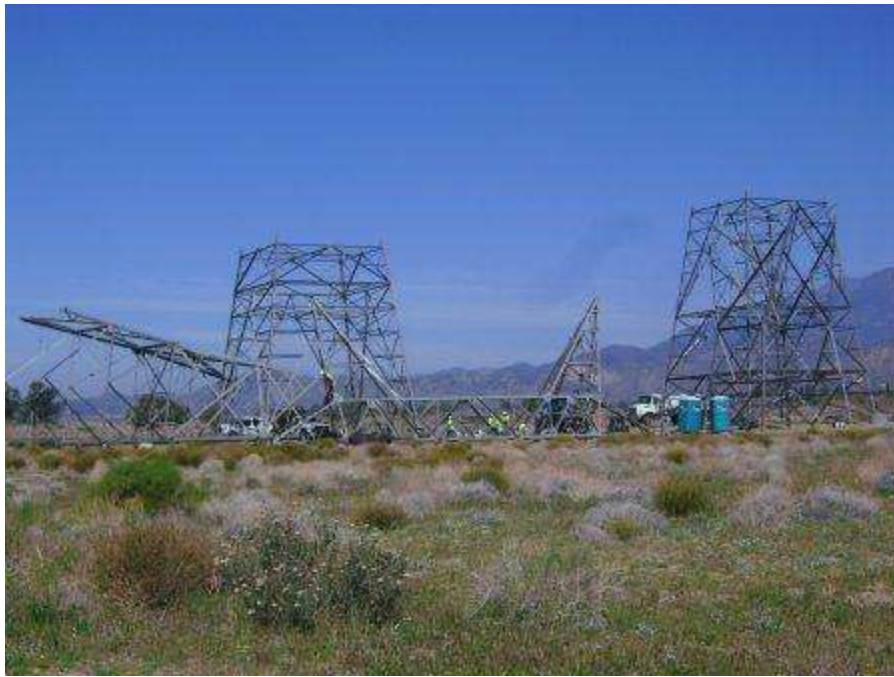
Figure 5. Tower assembly at Towers 1062 and R2.
