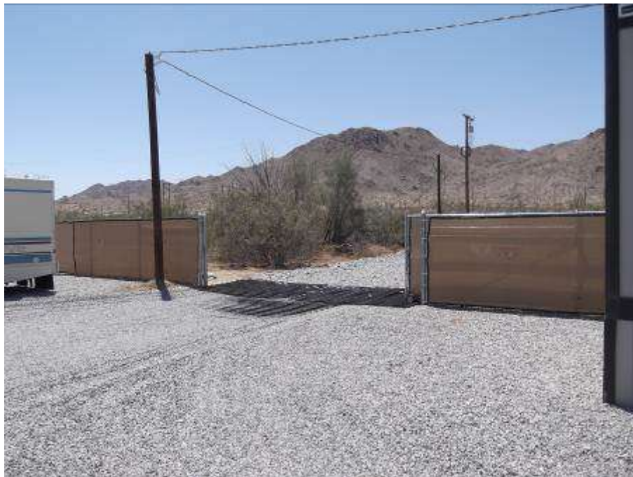
Figure 10. Entrance gate to the Chiriaco Summit Yard left open.
