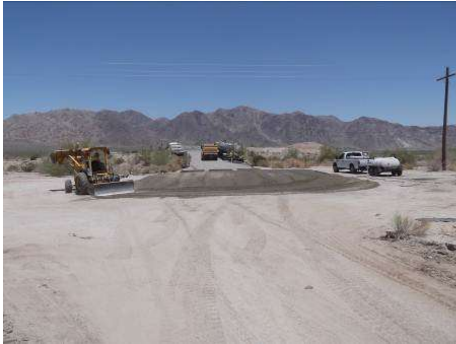
Figure 1. Installation of road base material at Hayfield Road.
