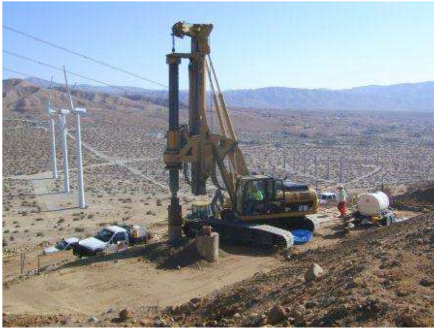
Figure 4. Foundation excavation drilling at Tower 1012.
