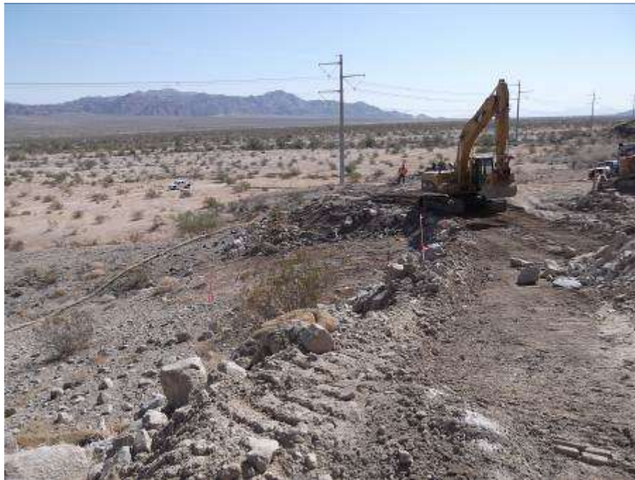
Figure 2. Vegetation clearing at Tower 2432.
