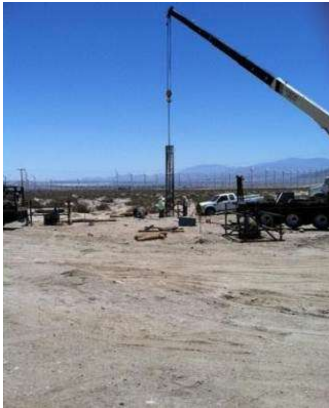
Figure 5. Rebar cage setting in preparation for concrete pour at Tower 1007.
