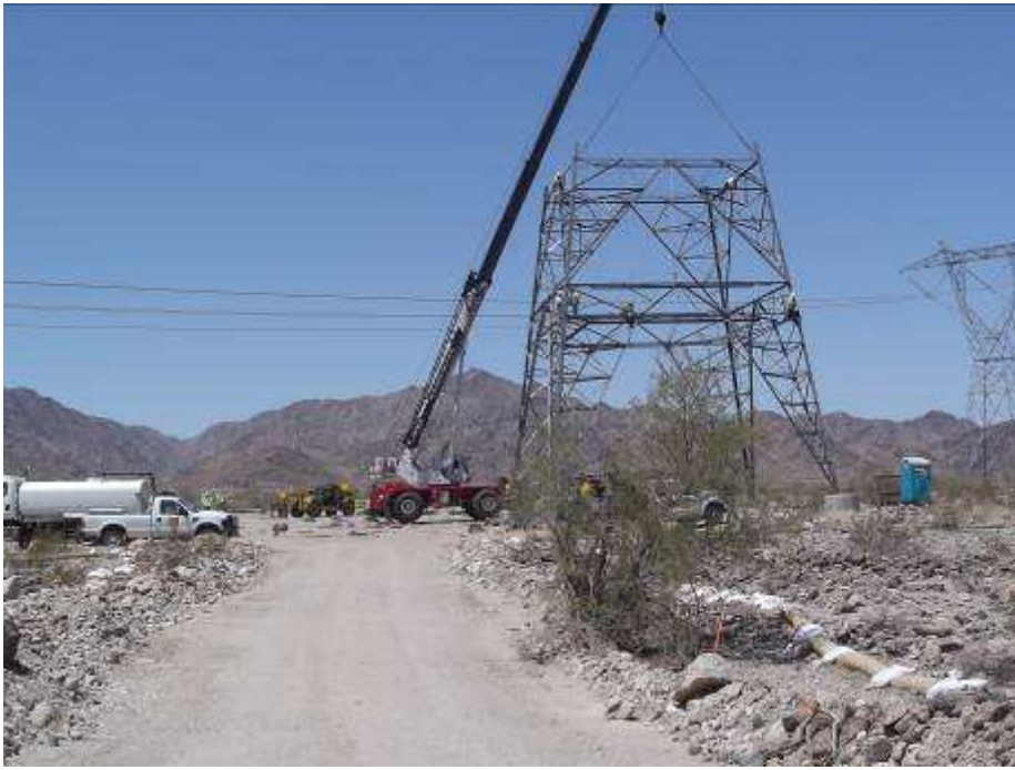
Figure 3. Tower assembly at RB2-5E.
