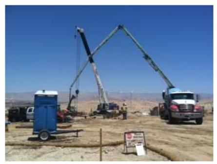
**Figure 1.** Foundation concrete pouring at Tower 2107
