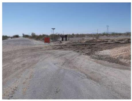
**Figure 7.** Excessive track-out identified at intersection of Chuckwalla and Corn Springs Roads.
