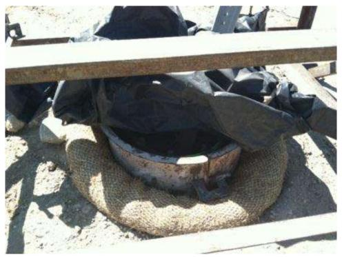
**Figure 3.** Inadequate covering of open excavation at Tower 1006.
