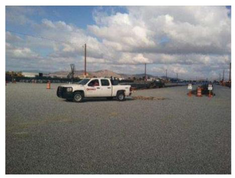
**Figure 10.** Contractor vehicle dragging a piece of fencing to comb gravel within the Menifee Yard.
