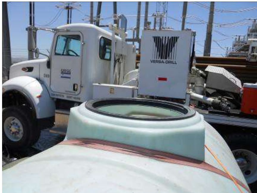
Figure 8. Water buffalo with no lid observed at Series Capacitor site.
