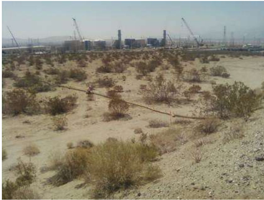
Figure 7. BMP installation for the Devers Substation Expansion Area.
