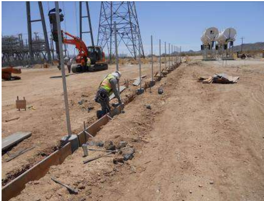
Figure 6. Fencing installation at Series Capacitor site.
