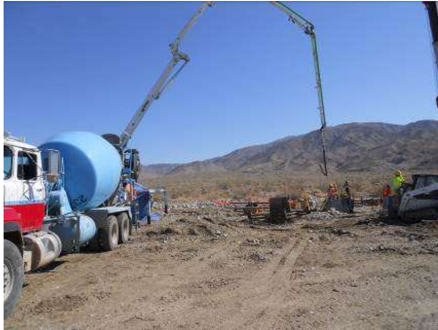
Figure 1. Concrete pouring occurring at Tower 2322.
