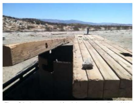
**Figure 5.** Inadequately covered foundation excavation at Tower 2015.
