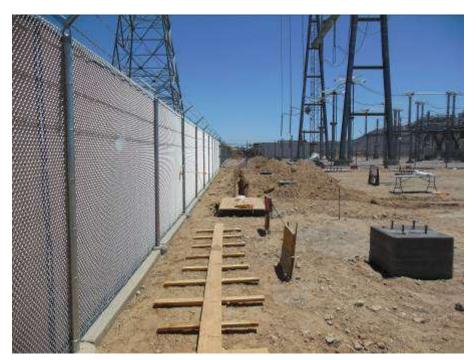
Figure 8. Trenching for ground wire installation at the Series Capacitor site.
