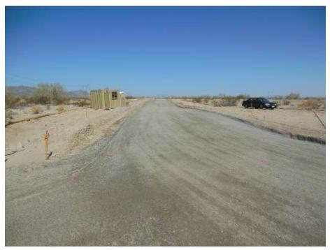
**Figure 9.** View west along Red Bluff access road where gravel road base has been installed.
