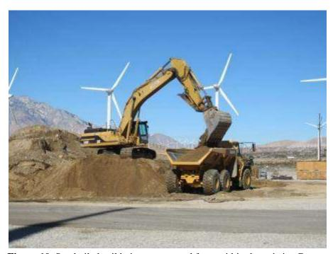
**Figure 10.** Stockpiled soil being transported from within the existing Devers Substation to the expansion area.
