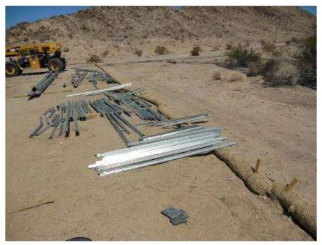
**Figure 7.** Tower hardware placed across BMPs at Tower 2409.
