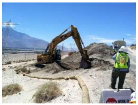
**Figure 1.** Excavating and grading activities for the spur road into Tower 2117.
