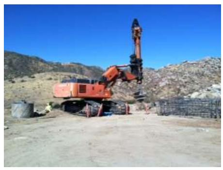
**Figure 3.** Foundation drilling activities at Tower 1071.
