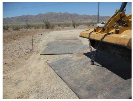
**Figure 2.** Installation of trench plates along the spur road to Tower 2415.
