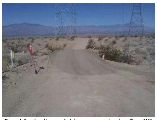
Figure 4. Gravel road base installed along an unapproved road near Tower 2303.
