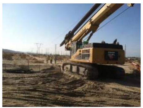
**Figure 4.** Drill rig being moved from Tower 2209 to Tower 2212 using both construction and biological monitor spotters to prevent off road impacts.
