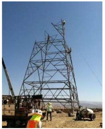
Figure 1. Tower assembly at Tower 2104.
