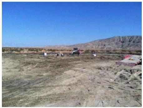
Figure 3. Grading for the spur road and crane pad at Tower 1003.
