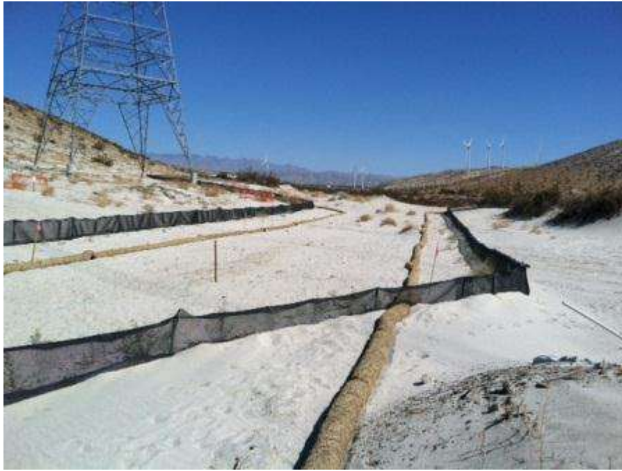
Figure 1. BMP installation at Tower 2110.
