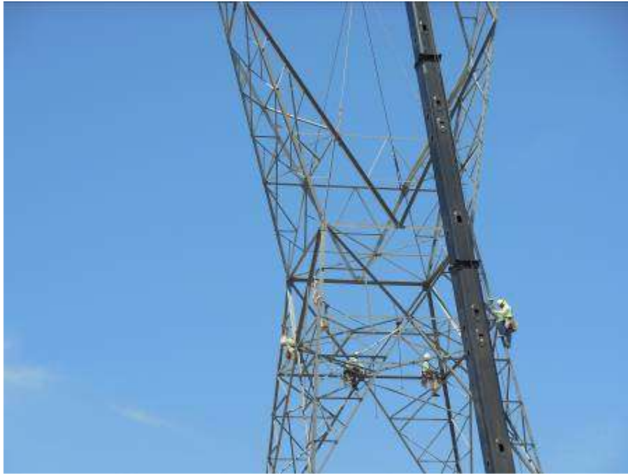
Figure 3. Assembly and erection activities at Tower 2522.
