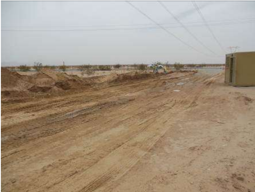
Figure 6. Grading activities along CRS access road.
