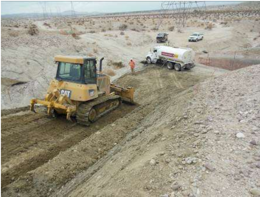
Figure 2. Grading the stub road at Tower 2233.
