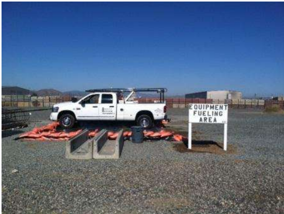
Figure 8. Containment areas established to ensure compliance at the Valley Substation.
