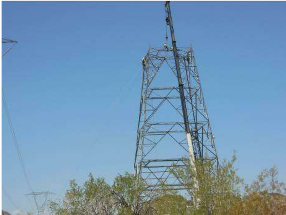
Figure 1. Assembly activities at Tower 2518.
