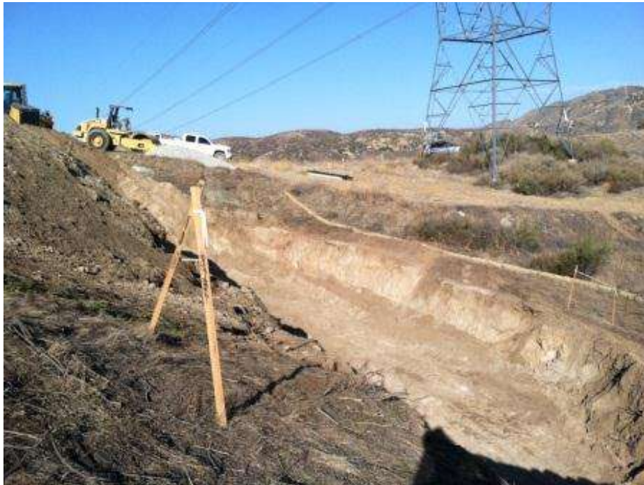
Figure 2. Grading activities at Tower 1110.
