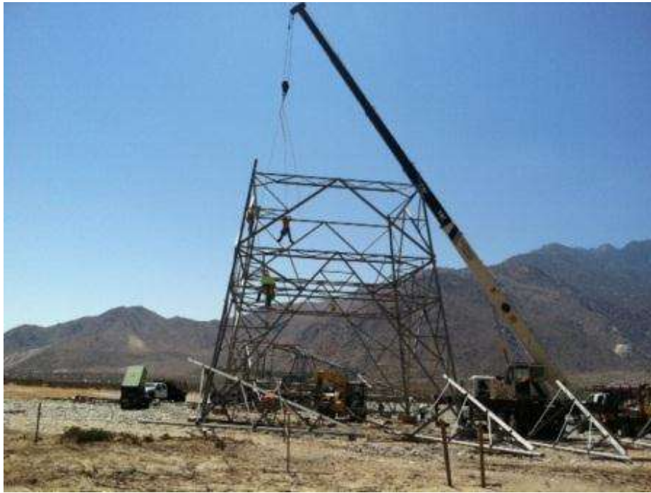
Figure 3. Tower assembly at Tower 1030.
