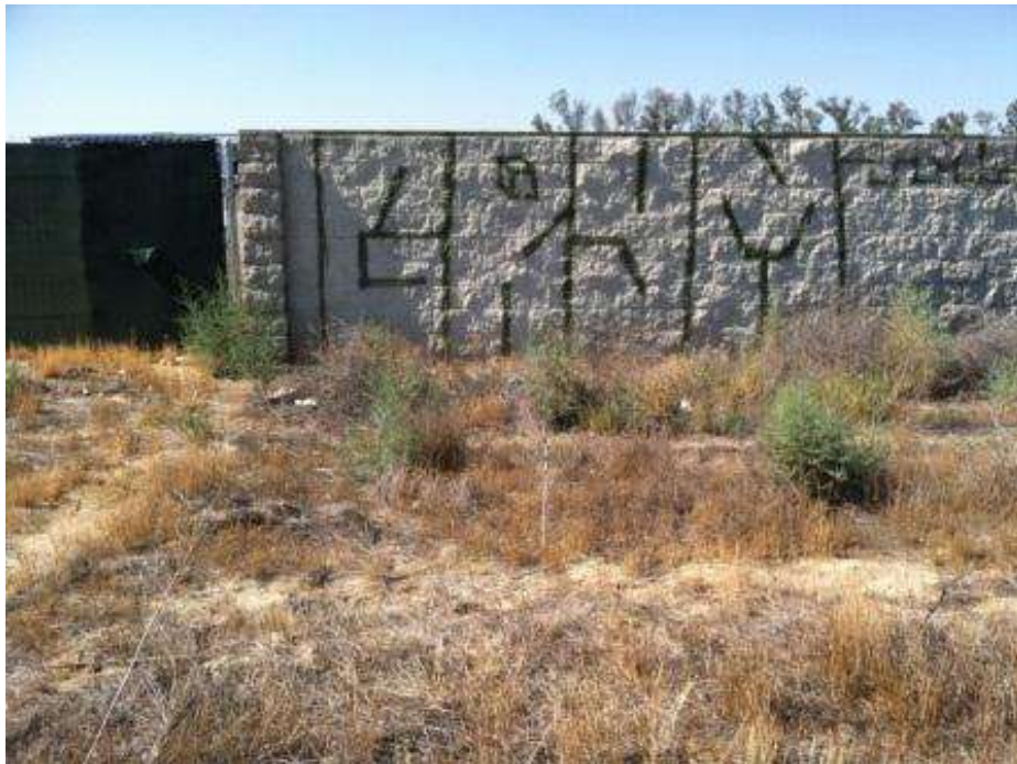
Figure 10. Graffiti discovered of the wall at the Perris Yard. Photo courtesy of FRED.
