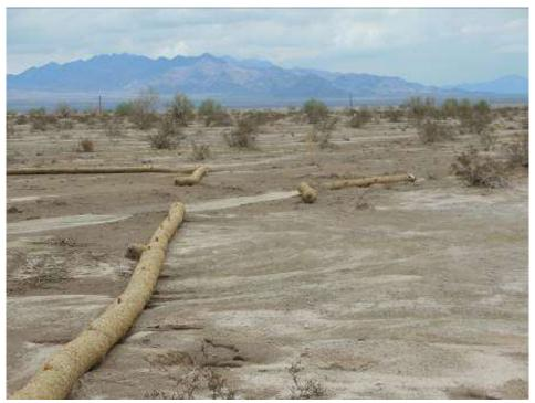
Figure 6. Storm damage to BMPs at Tower 2608.
