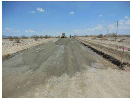
Figure 9. Road base installation continued along the Red Bluff access road.
