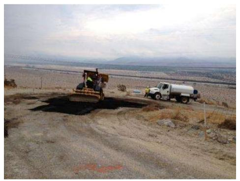
**Figure 2.** Asphalt repair on the access road to Tower 2117. (Photo Courtesy of FRED)
