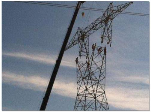
Figure 4. Tower Bridge erection at Tower 2127.
