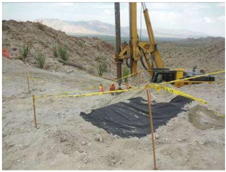
Figure 7. Properly covered foundation excavation at Tower 2547.
