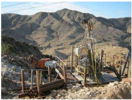
Figure 3. Micropile drilling at Tower 2424.
