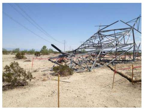
**Figure 8.** Tower section that had fallen over due to inclement weather and partially landed outside the disturbance limits at Tower 2538. Photo courtesy of FRED report.
