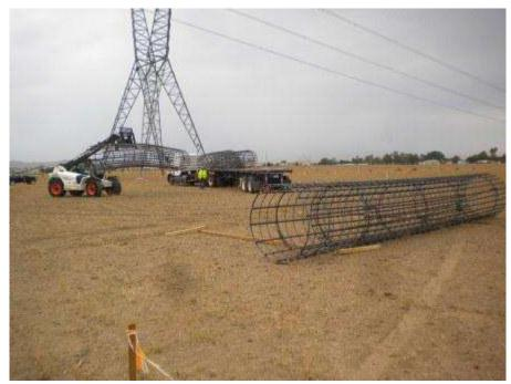
Figure 9. Delivery of rebar cages to Tower 1155 prior to the site being released to SCE. Photo courtesy of FRED report.
