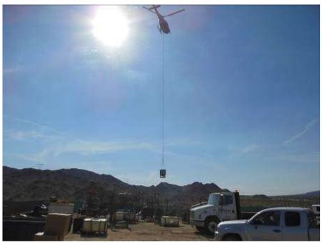
Figure 3. Transfer of grout from hopper to bucket at HLZ H5 for micropile activities at Tower 2424.
