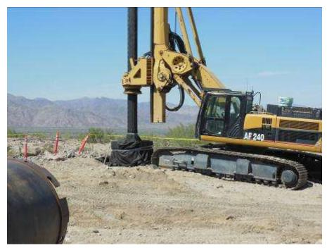
Figure 10. Partially excavated foundation with adequate covering at Tower 2507.
