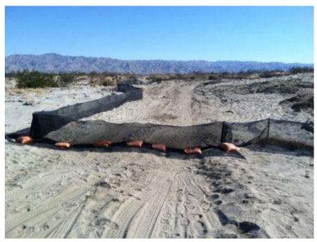
Figure 5. Repairs to Coachella Valley Fringe-toed Lizard exclusionary fencing completed at Tower 2013.
