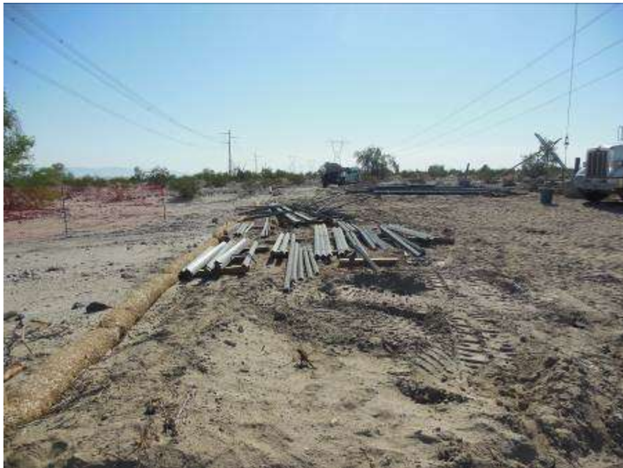
Figure 7. Steel material staged across straw wattle BMPs at Tower 2543.
