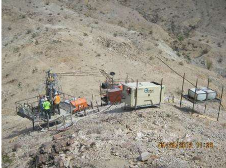
Figure 2. Micropile foundation drilling activities at Tower 2309.
