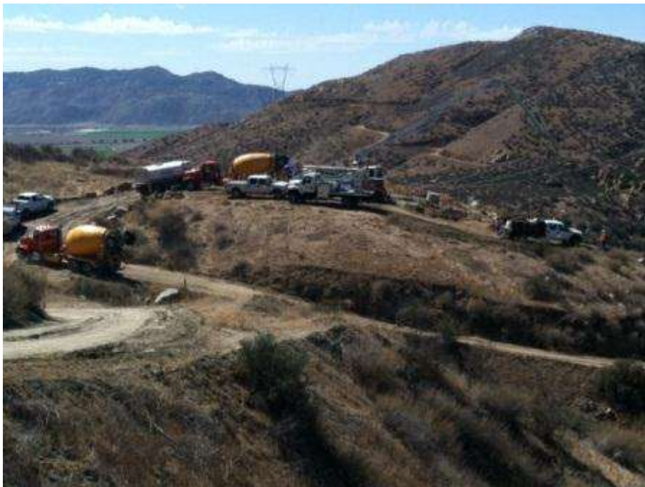
Figure 6. Tower foundation concrete pouring activities at Tower 1111.
