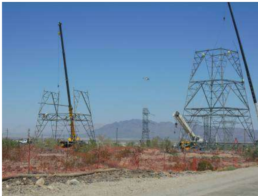
Figure 4. Assembly crews onsite at Towers RB1-2W and RB2-2W.
