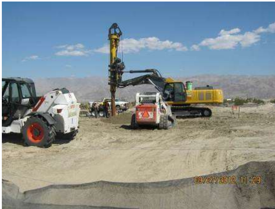
Figure 3. Foundation drilling activities at Tower 2242.
