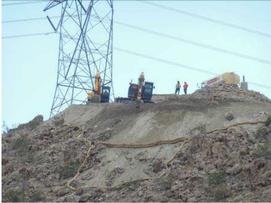
Figure 1. Grading activities at Tower 2416.
