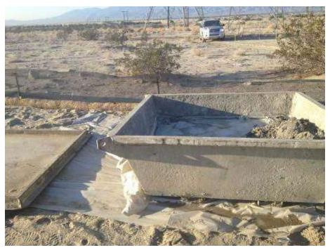
Figure 5. Eco-pan was left uncovered at Tower 2242. Photo courtesy of FRED.
