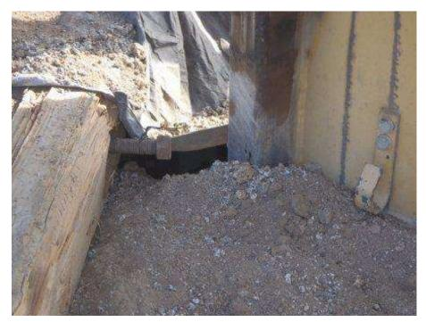
Figure 7. Partially uncovered hole discovered at Tower 1148.
