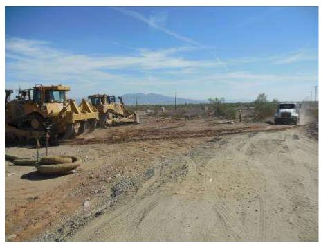
Figure 1. Grading activities at Guard Structure RB-GS06.
