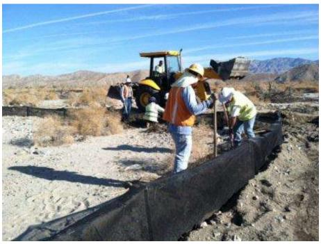
Figure 3. Installation of Coachella Valley Fringe-toed Lizard exclusionary fence at Wire Site 14/ Pull Site 15.
