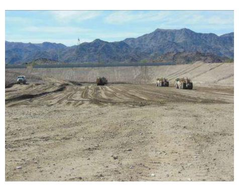
Figure 8. Backfilling of the drainage basin at Red Bluff Substation.
