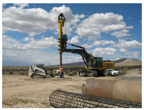
Figure 3. Foundation drilling at Tower 2306.
