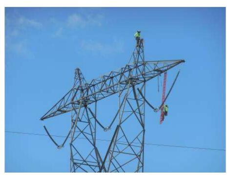
Figure 4. Installation of insulators at Tower 2543.
