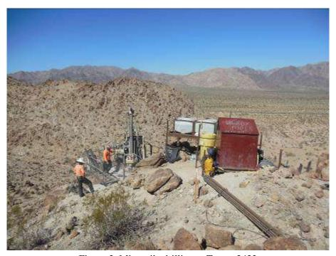
Figure 2. Micropile drilling at Tower 2422.
