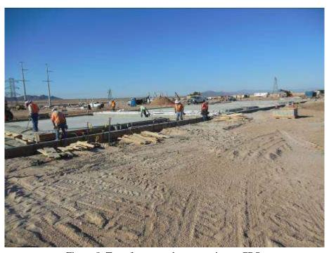
Figure 8. Transformer pad construction at CRS.
