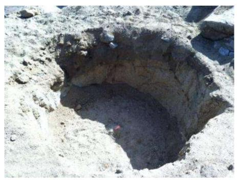
Figure 8. Uncovered steep-walled excavation at Tower 1036 that resulted in NCR #11.
