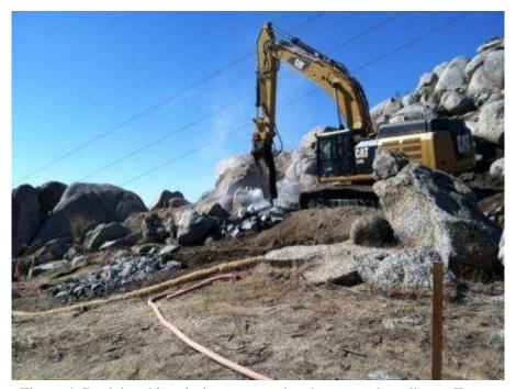
Figure 4. Rock breaking during spur road and crane pad grading at Tower 1127.
