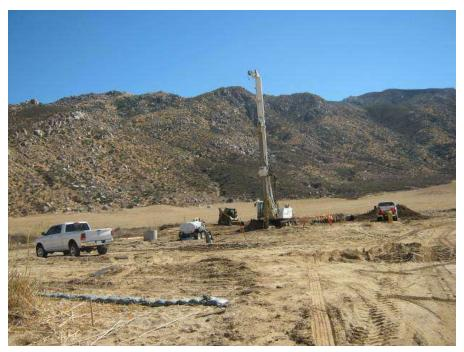
Figure 7. Foundation drilling at Tower 1084.
