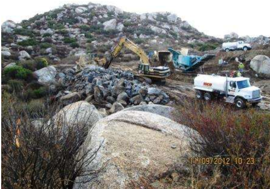
Figure 4. Grading and rock crushing activities at Tower 1142.
