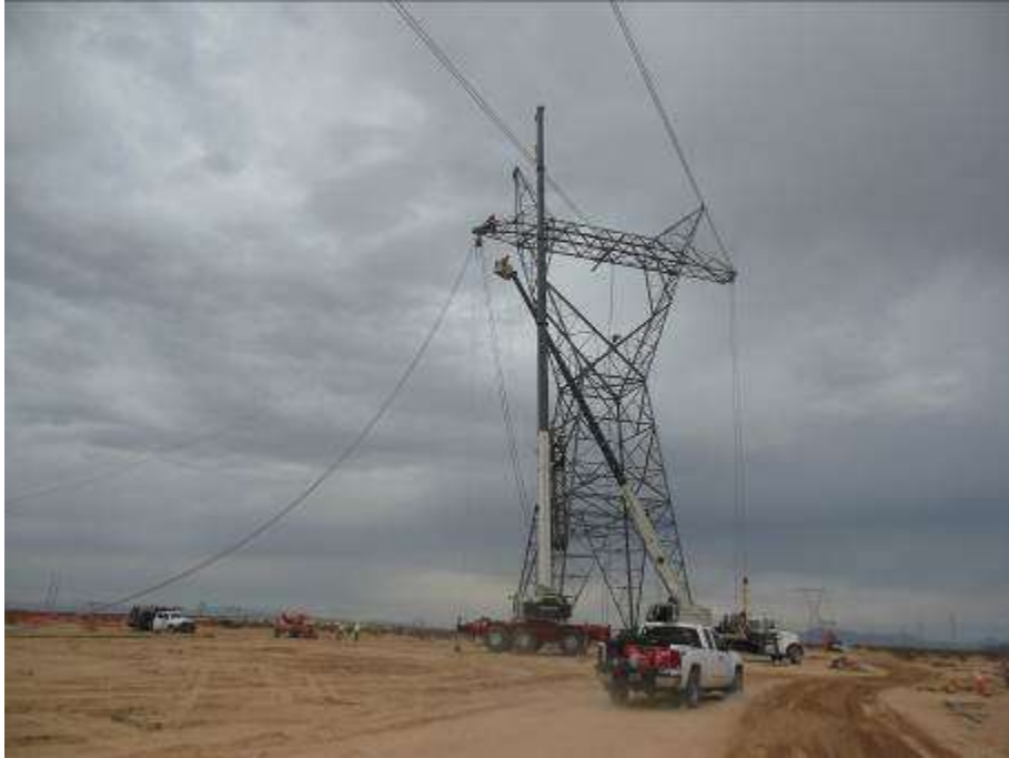
Figure 1. Stringing activities at CR1-5E and associated wire stringing sites.
