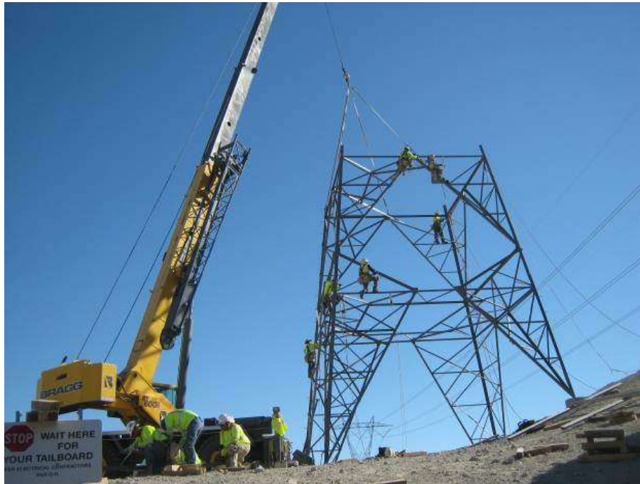
Figure 2. Assembly and erection at Tower 2415.
