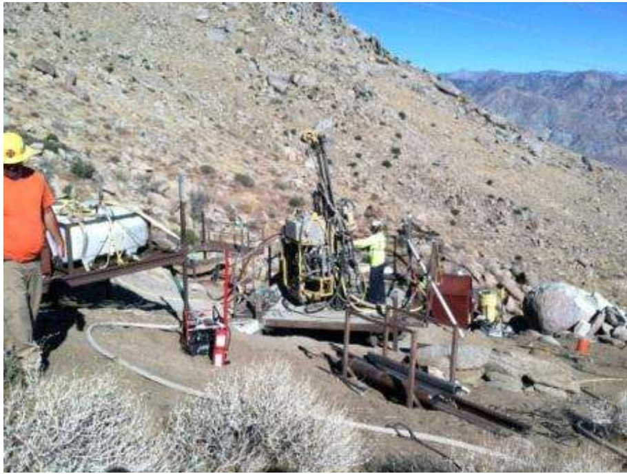
Figure 5. Micropile drilling activities at Tower 1037.
