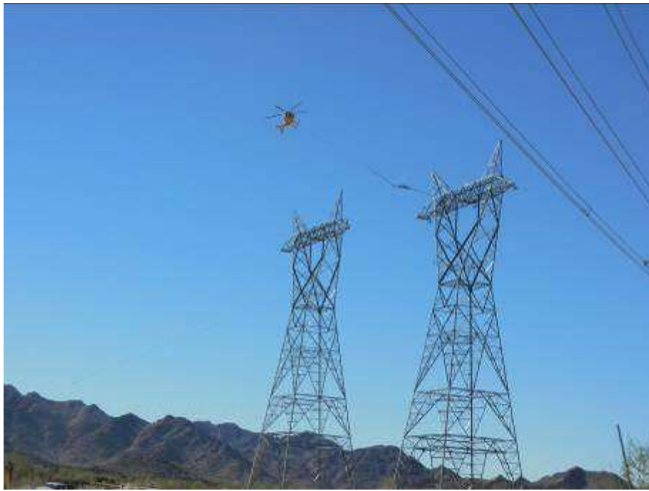
Figure 3. Pulling sockline at the Red Bluff loop-in towers.
