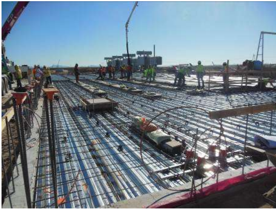
Figure 9. Construction of the basement ceiling for the MEER building at CRS.
