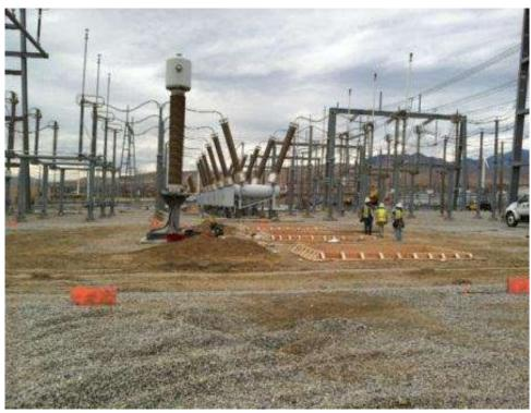
Figure 9. Foundation work for the 500 kV switchrack within the Devers Substation expansion.
