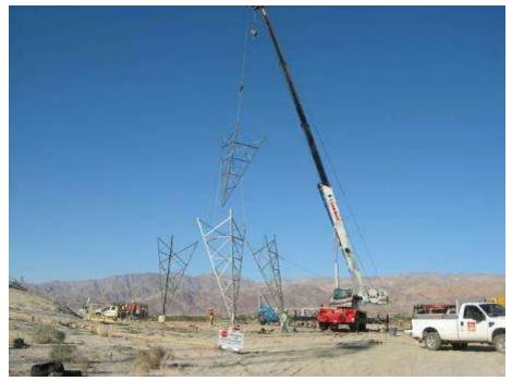
Figure 3. Steel erection at Tower 2246.
