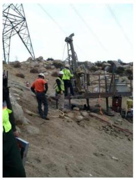
Figure 4. Micropile drilling at Tower 1038.
