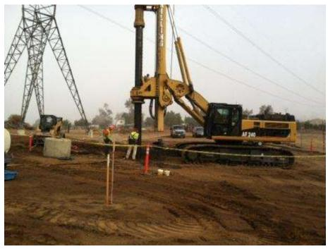
Figure 5. Foundation drilling at Tower 1147.
