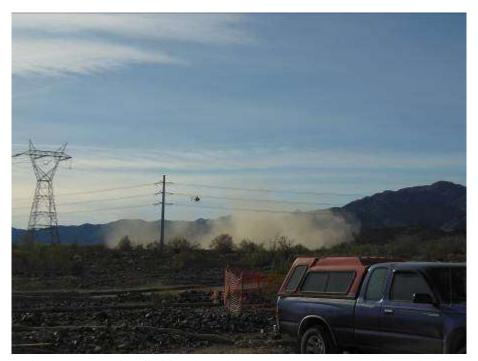
Figure 8. Excessive fugitive dust observed by CPUC EM during stringing activities at Wire Site RB-03.
