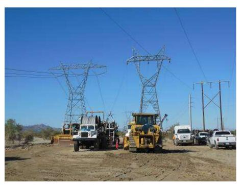
Figure 1. Set up of wire stringing equipment at Wire Site 77.
