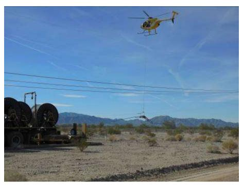
Figure 4. Wire stringing activities between the Red Bluff loop-ins and Tower 2539.
