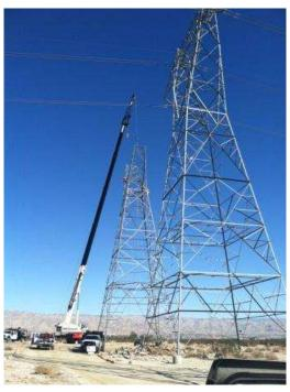
Figure 3. Tower assembly at Tower 2008.
