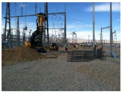
Figure 9. Foundation excavation for the 500 kV Switchrack within the Devers Substation.
