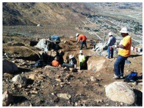
Figure 5. Micropile site preparation at Tower 1050.
