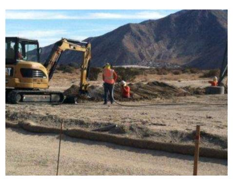
Figure 6. Ground wire trenching at Tower 1024.
