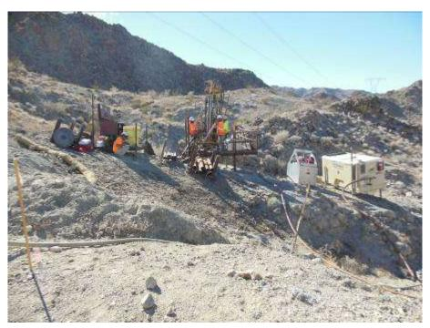
Figure 2. Micropile drilling at 2421.
