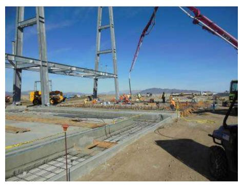
Figure 10. Transformer pad and switchrack construction at Red Bluff Substation.
