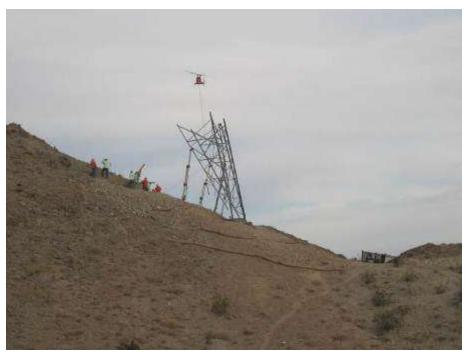
Figure 3. Micropile steel erection at Tower 2308.
