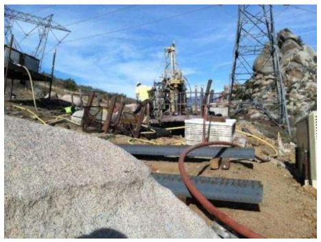
Figure 7. Micropile drilling on USFS site Tower 1040.
