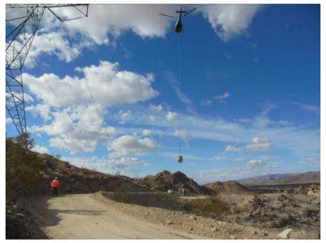
Figure 2. Installation of grout at micropile Tower 2421.
