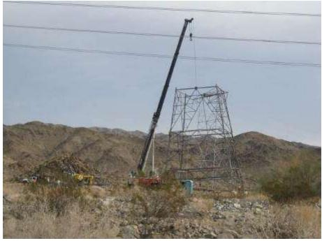
Figure 3. Steel erection at Tower 2326ALT.
