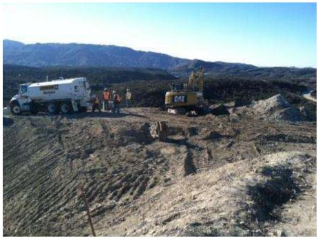
Figure 5. Crane pad grading at Tower 1097.
