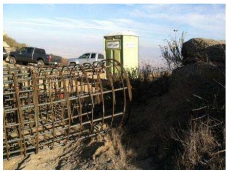
Figure 6. Steel rebar cages extending outside of the approved disturbance area at Tower 1127.
