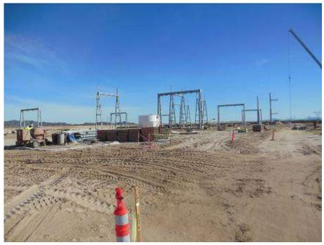
Figure 7. Assembly and installation of switchracks at CRS.
