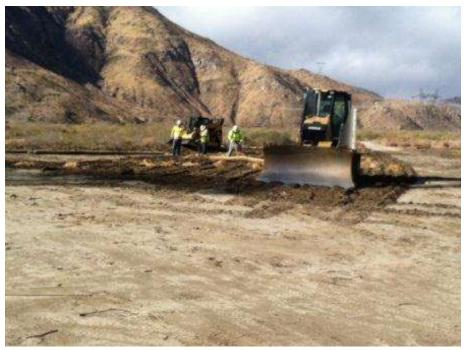
Figure 4. Restoration activities at Pull Site R2, including grading and BMP removal.
