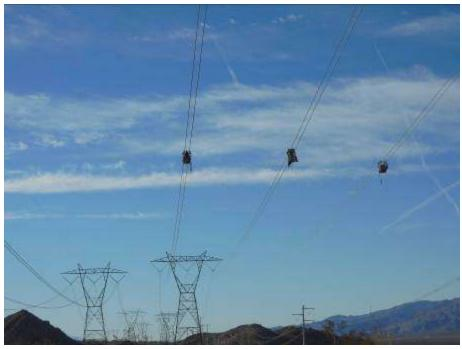
Figure 3. Installing spacers between Towers 2503 and 2504.
