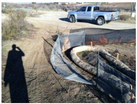
Figure 5. Damaged SKR exclusionary fencing at Tower 1133.
