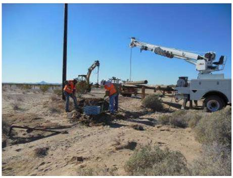
Figure 6. Hole excavation for wooden pole installation along the Southeast Telecommunication Route.
