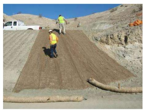
Figure 1. Installation of jute netting on slope at Tower 2238.
