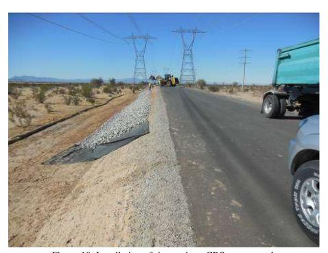
Figure 10. Installation of riprap along CRS access road.
