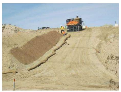
Figure 2. BMP jute netting installation on side slope at Tower 2234.
