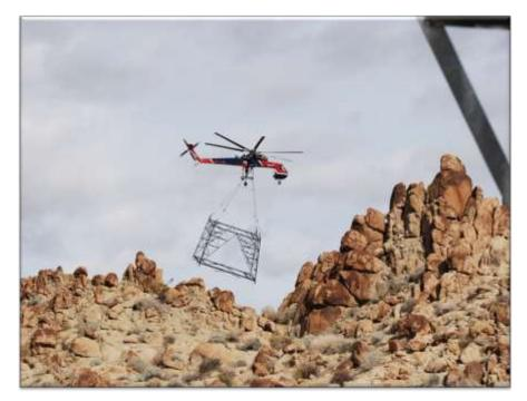
Figure 4. Transporting tower laybacks to Tower 2425 via Skycrane.
