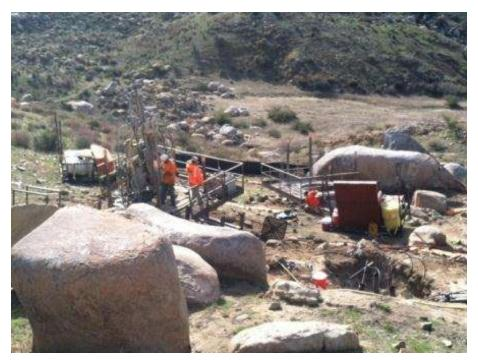
Figure 6. Micropile drilling at Tower 1074.
