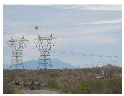
Figure 2. Pulling sockline at Tower 2327.
