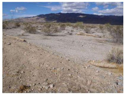
Figure 7. Straw wattle BMPs requiring maintenance at Tower 2332 (photo courtesy of FRED).
