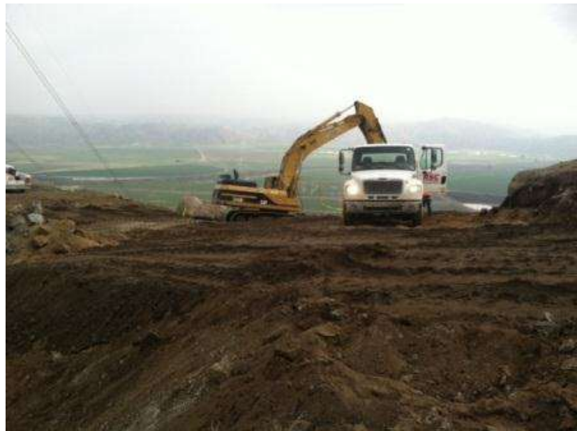
Figure 6. Grading activities at Tower 1123.
