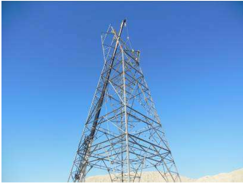
Figure 3. Erection of laybacks at Tower 2226.
