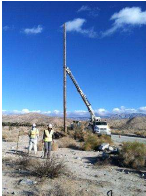
Figure 2. Guard pole installation near Tower 2202.
