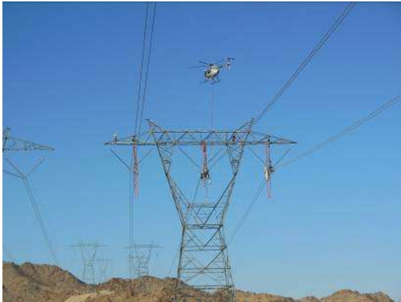
Figure 4. Clipping conductor at Tower 2426.
