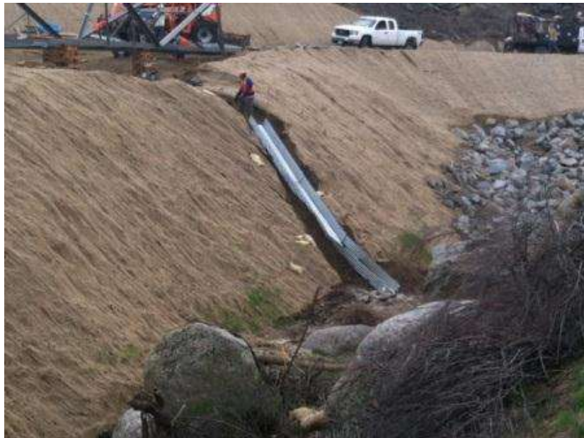
Figure 8. Installing drainage system at Tower 1141.
