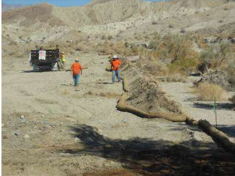
Figure 1. Topsoil salvage at Pull Site 24.
