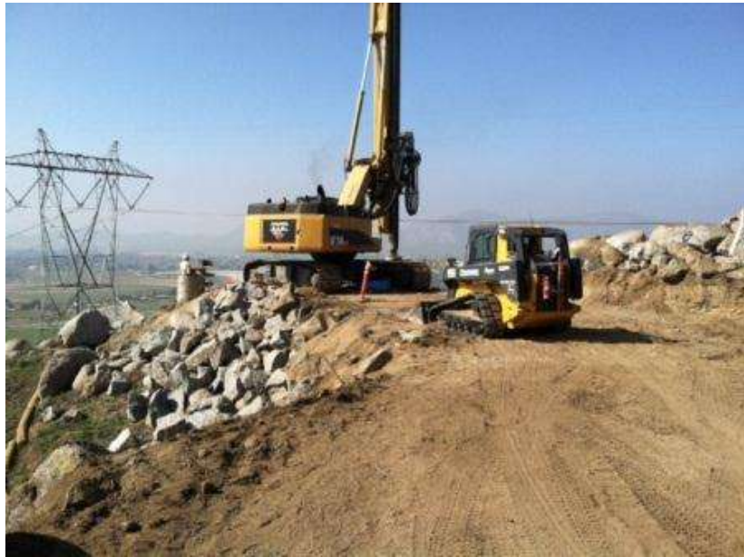
Figure 7. Foundation drilling at Tower 1131.
