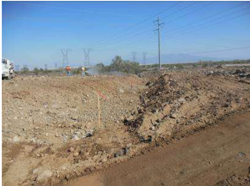
Figure 5. Recontouring of drainage through Wire Site RB-01.
