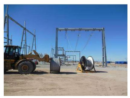
Figure 8. Stringing wire along switchrack at CRS.
