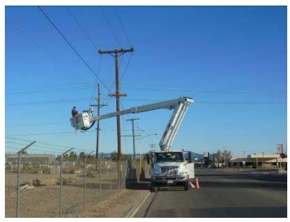
Figure 9. Wire stringing from bucket truck along SE Telecomm line.
