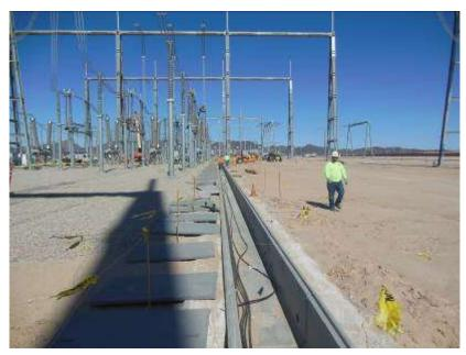
Figure 7. Installation of conduit at CRS.
