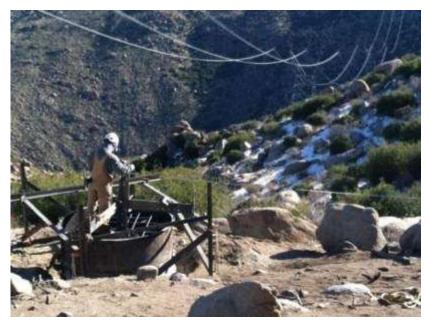
Figure 5. Pilecap preparation at Tower 1044.
