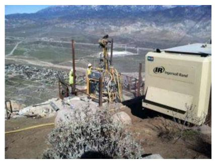
Figure 3. Micropile drilling at Tower 1049.
