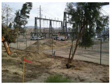
Figure 9. Trenching activities for the Mirage Loop-ins inside and outside of the Mirage Substation.
