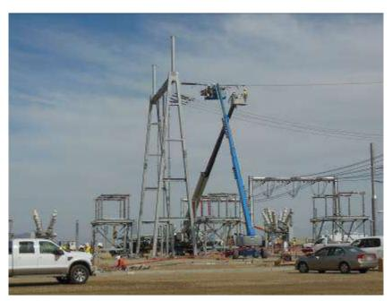
Figure 8. Wire stringing at Red Bluff Substation.
