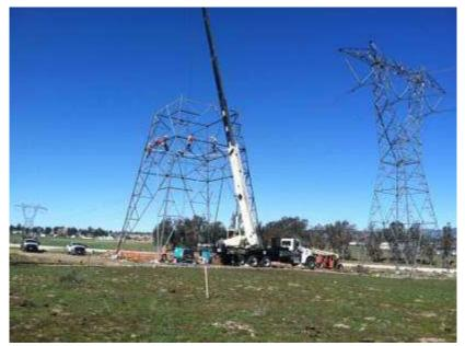
Figure 5. Tower assembly at Tower 1077.
