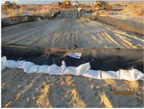
Figure 6. CVFTL fencing damaged at Wire Site 27. Photo courtesy of FRED.
