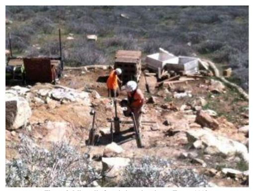
Figure 2. Micropile foundation trimming at Tower 1112.
