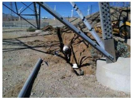
Figure 8. Telecommunications conduit trench work from the Devers Substation to Tower 1000X.
