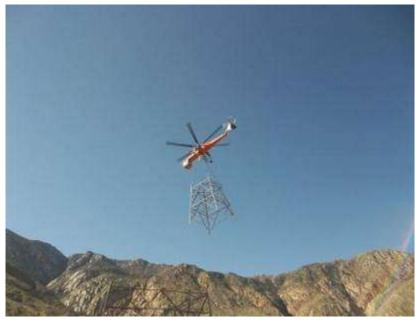
Figure 3. Skycrane lifting a tower section out of HLZ H2. (Photo courtesy SCE).
