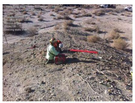
Figure 4. OPGW crew conducted sleeving of the static wire outside the approved disturbance areas between Towers 2230 and 2230AX. (Photo courtesy of FRED)
