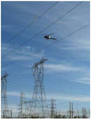
Figure 3. Traveler and insulator installation by helicopter at Tower 1003.
